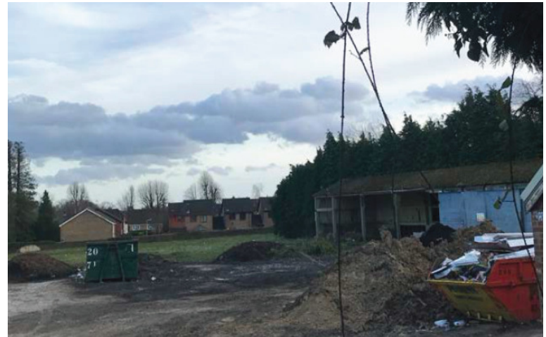
(internal view facing south)
