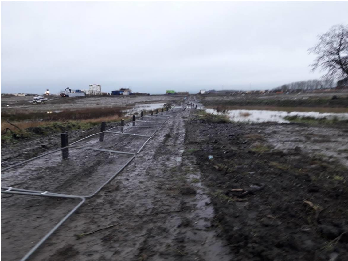
Plate 12: Overview of old road with flooding at either side, taken from TP363 looking north.
