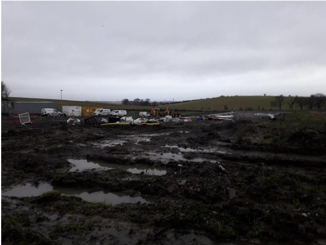
Plate 3: Overview of earthworks and existing site compound in the northern field.
