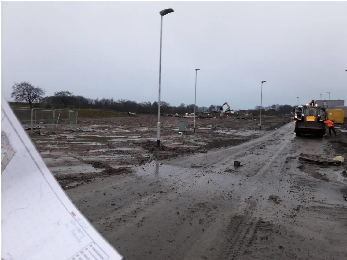
Plate 6: Overview of earthworks in the northern field.
