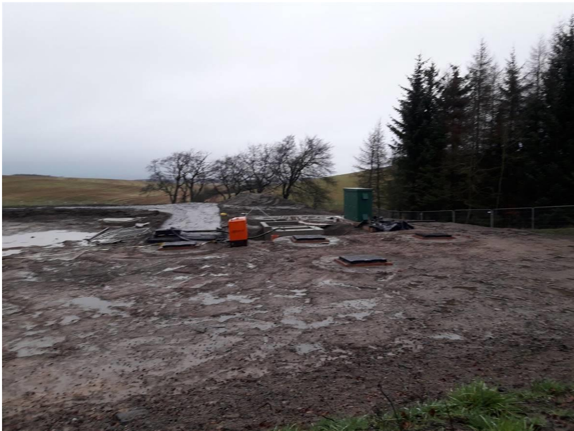
Plate 4: Overview of earthworks in the eastern boundary of northern field.
