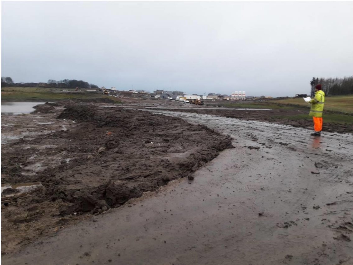
Plate 5: Overview of earthworks in the northern field.
