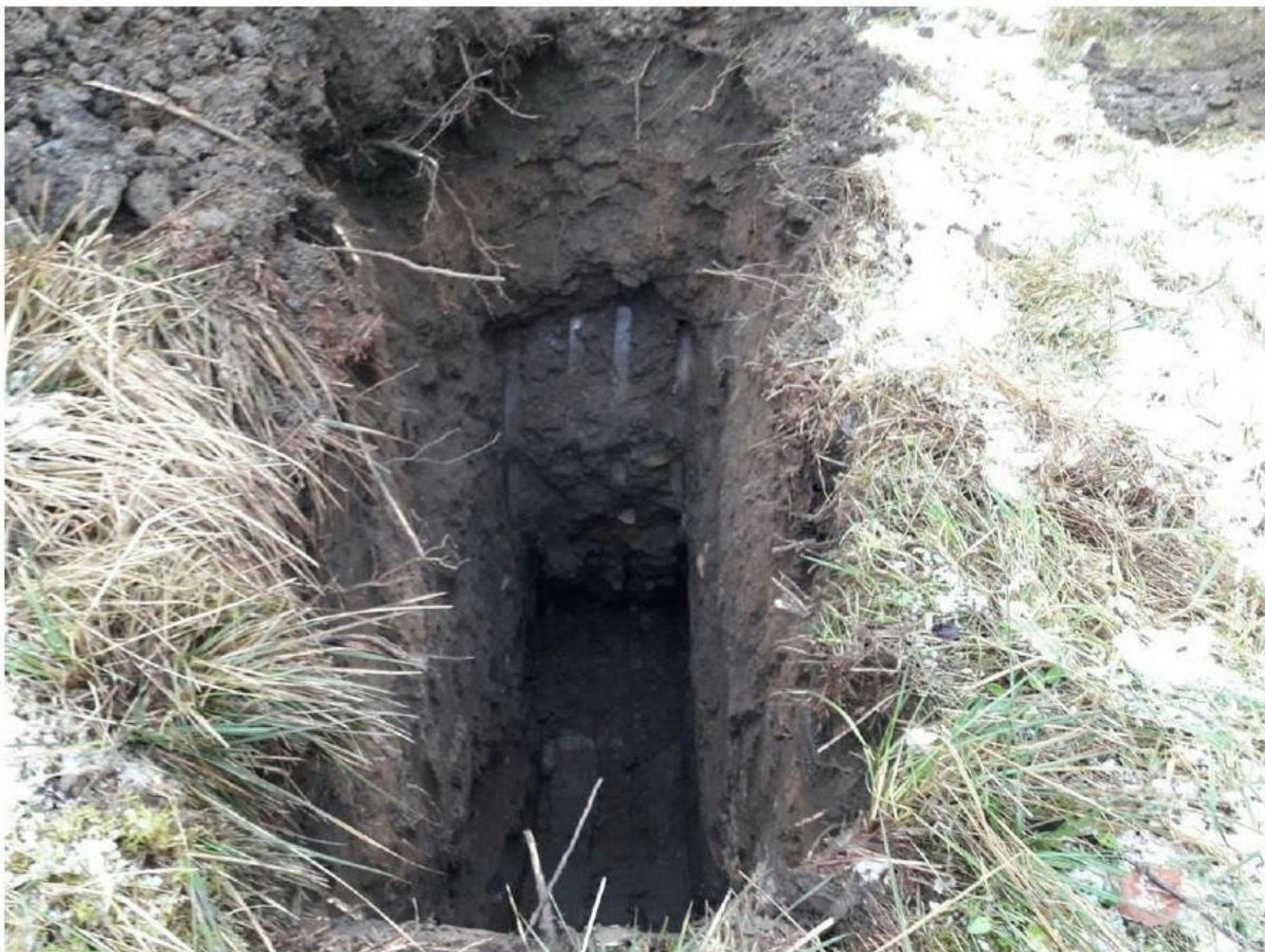
Plate 44: Detailed view of sidewalls of completed TP387.
