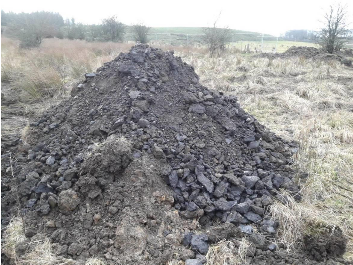
Plate 23: Overview of excavate material at TP327.
