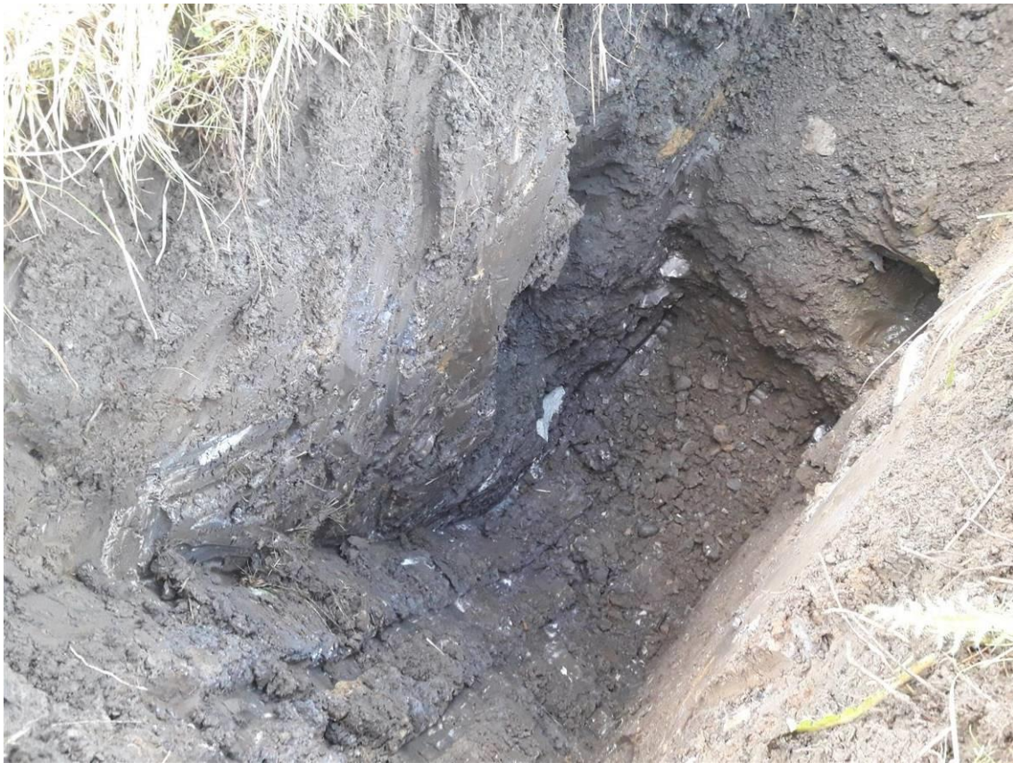
Plate 18: Detailed view of sidewalls in completed TP302.
