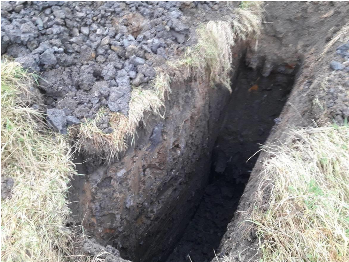
Plate 30: Detailed view of sidewalls in completed TP346.
