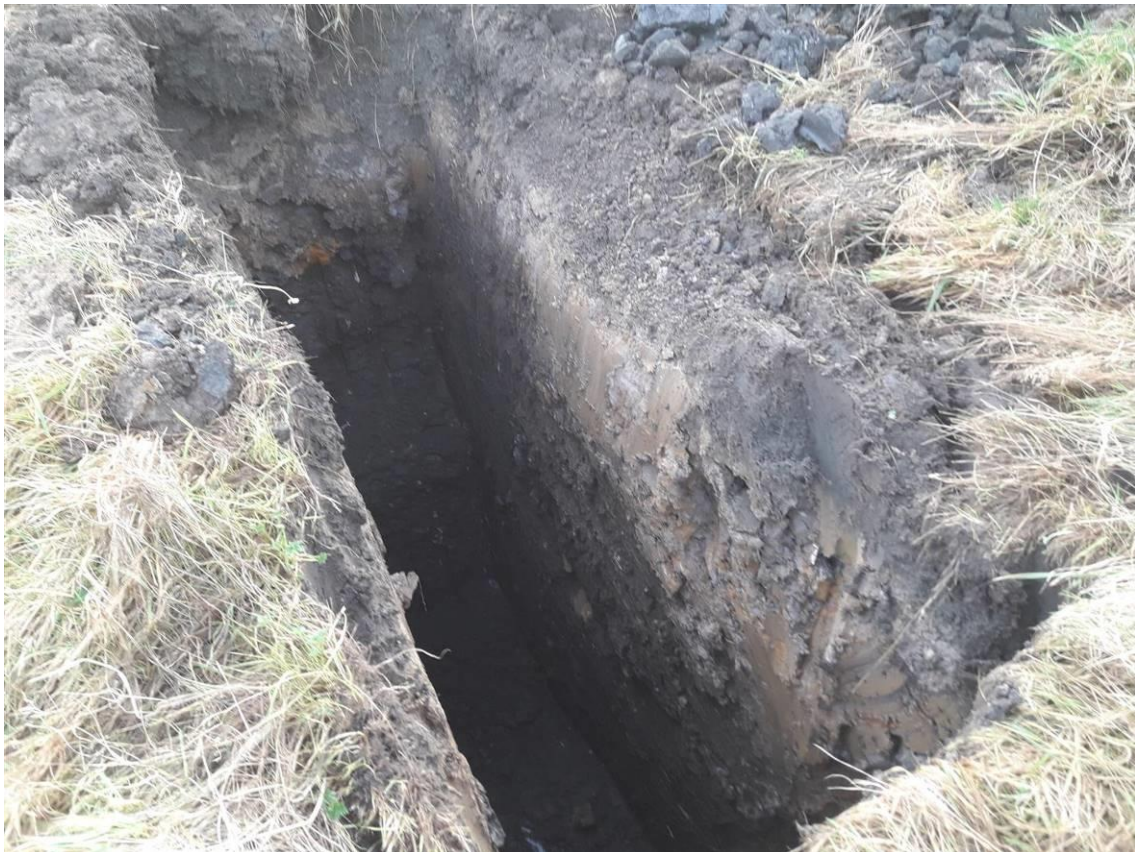
Plate 26: Detailed view of sidewalls in completed TP334.
