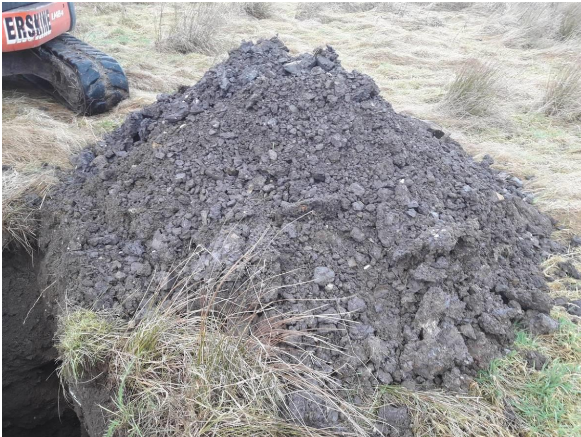
Plate 17: View of excavated material from TP302.
