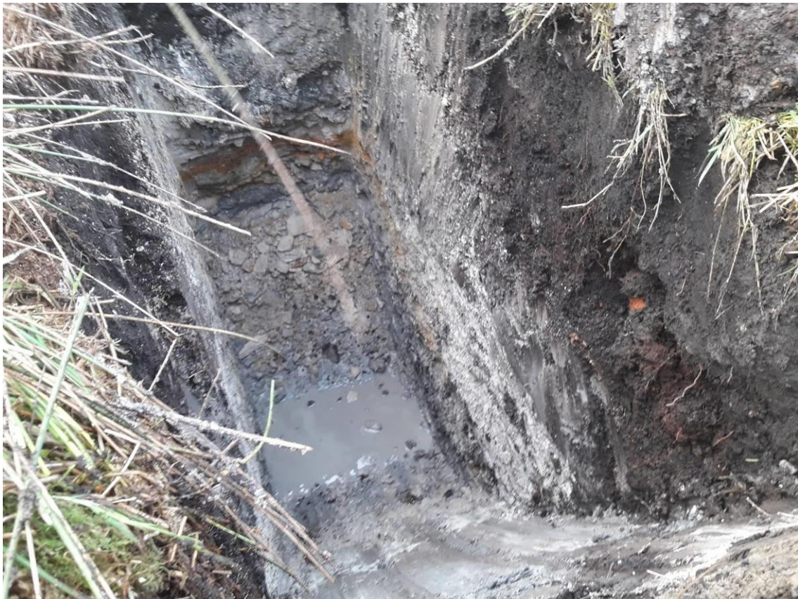
Plate 20: Detailed view of sidewalls in completed TP311.
