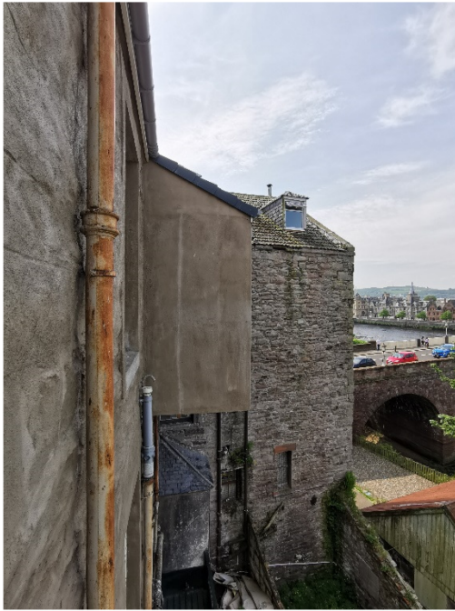
Figure 5 – timber vestibule at rear
