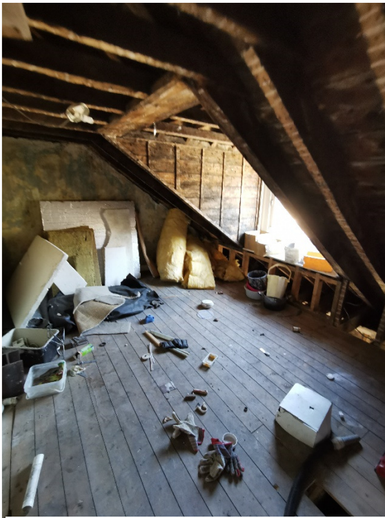
Figure 1 – upper floor (at dormer)
