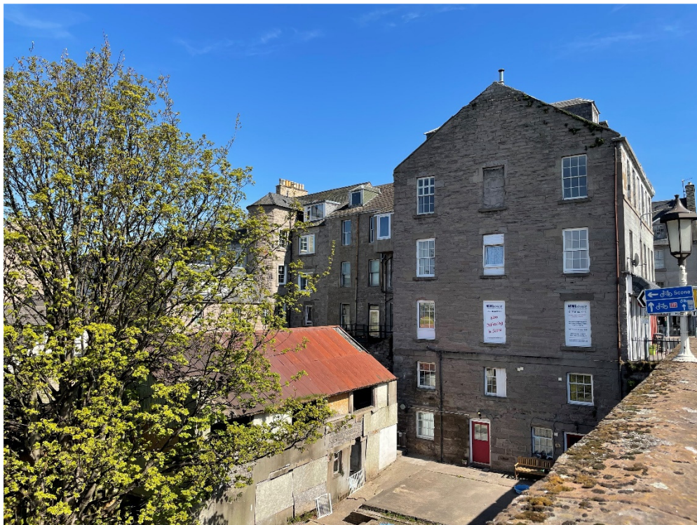
Figure 7 – rear elevation from bridge
