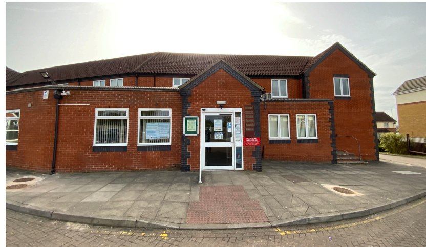
View of the Main (rear) Entrance.
