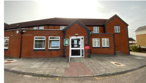
View of the Main (rear) Entrance.
