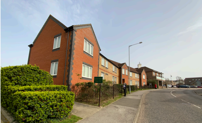
View looking South East, at the Road-Facing Facade
