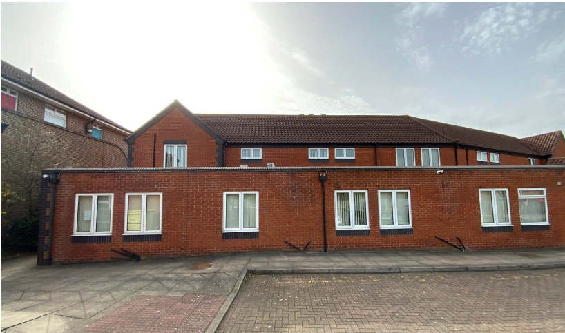
View over the existing rear flat-roof wing (foreground) and First floor administration accommodation (background).
