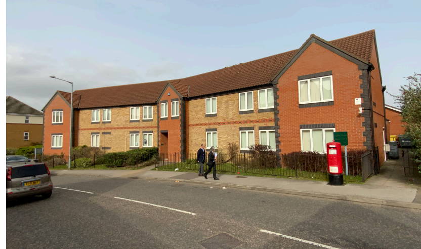
View looking North East, at the Road-Facing Facade
