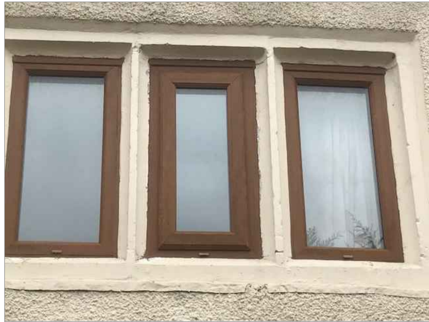
W1 - Window to be replaced
