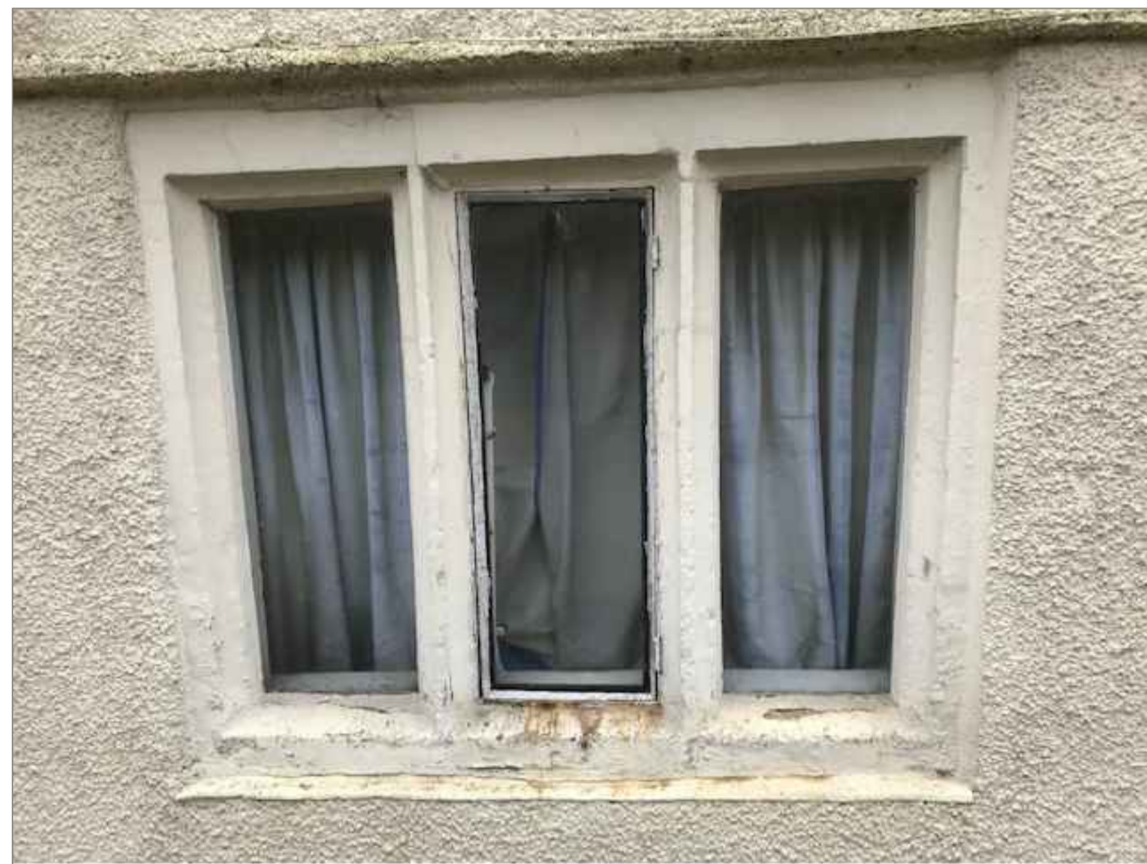
Example of original Crittall Steel Windows on the same property
