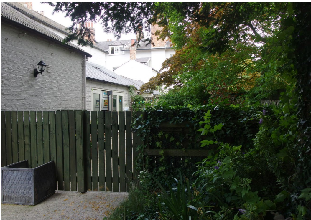
image b - the 21st century infill to the ancillary buildings and separate external space to Magnolia Cottage. The main house is visible behind.
