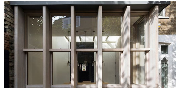
Example glass extension - large amounts of glazing reveal the heritage asset behind while the vertical emphasis and proportions tie in; timber softens
