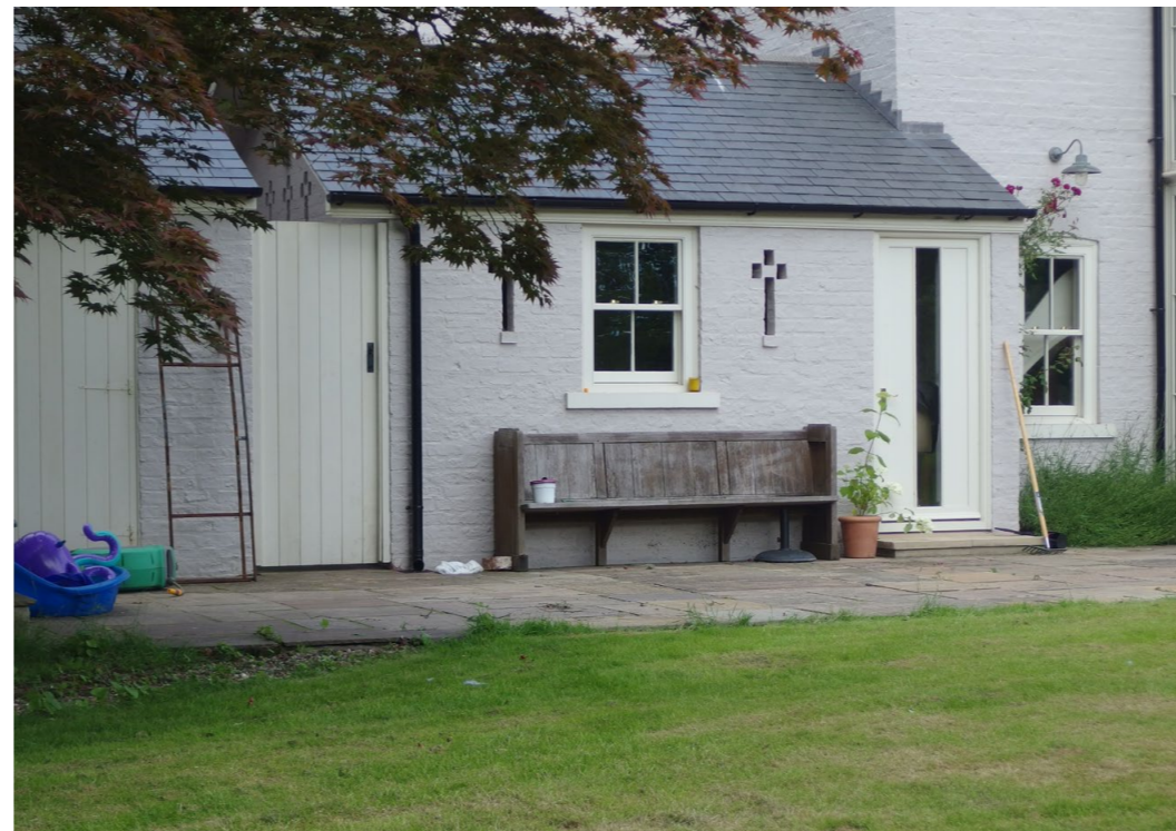
image c - the east elevation to the chapel - the distinction between the main house and ancillary buildings is reduced by the solid gate between the chapel and store
