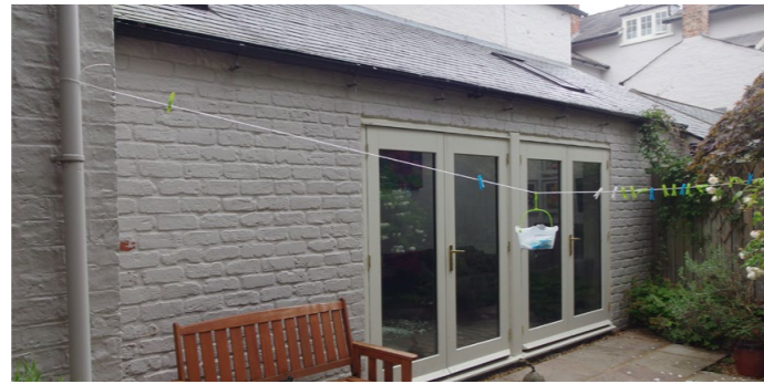
21st century infill to ancillary buildings - connecting views are blocked by current landscaping
