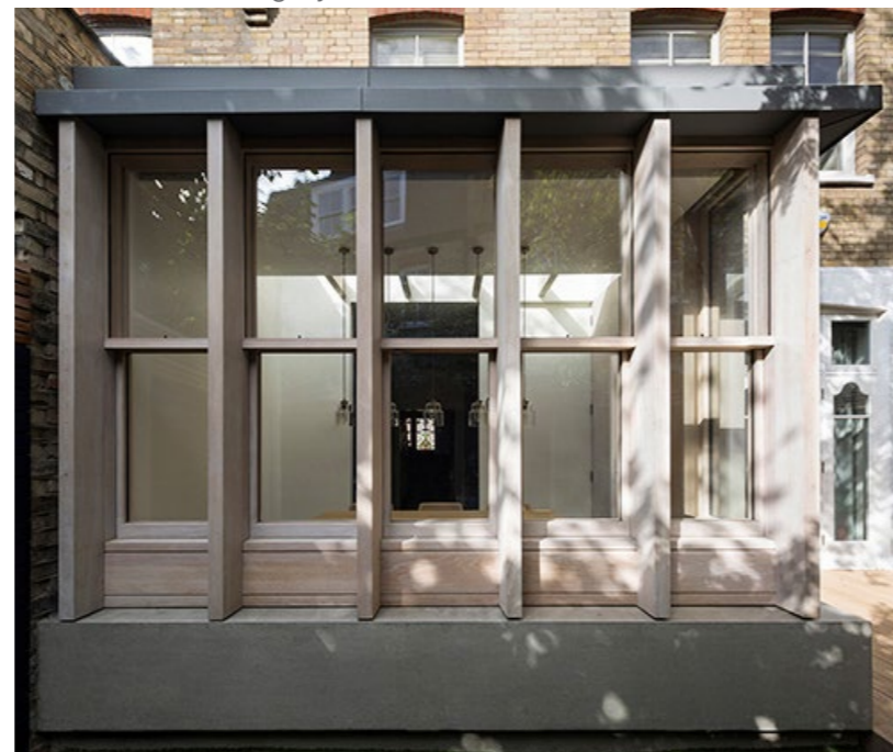
Belsize House extension by Studio Carver
