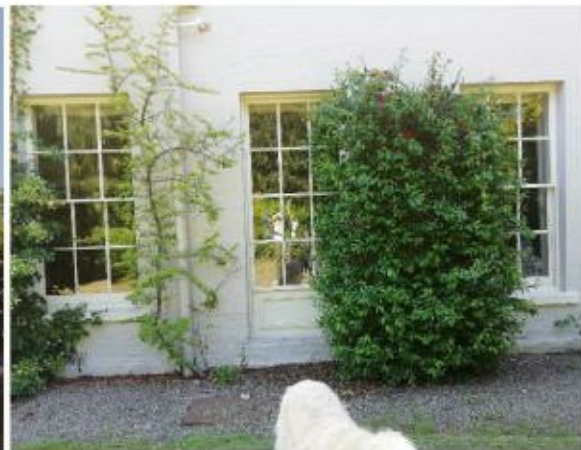
Fig 13 C18th central doorway now blocked
