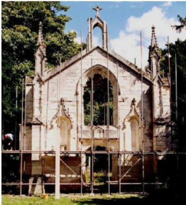
Fig 28 Scaffold erected to demolish west face
