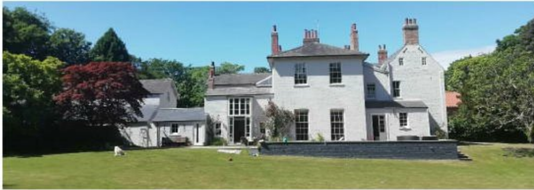
Fig 15 East elevation with C18th gable to right and C19th and C21st extensions to left
