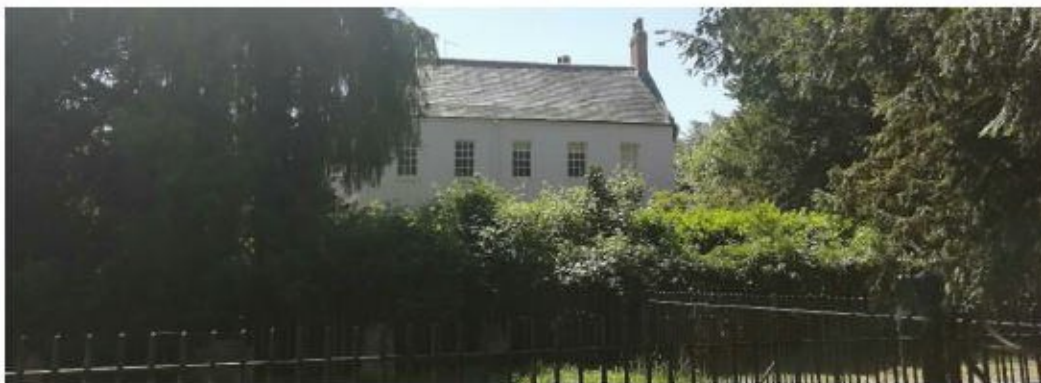
Fig 18 Ground floor of original, principal elevation of C18th dwelling concealed by hedge
