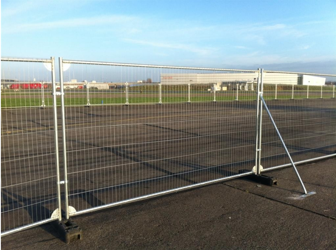
Figure 4: Secured 'Heras' type fencing with stabilizing system and anti-tamper couplers
