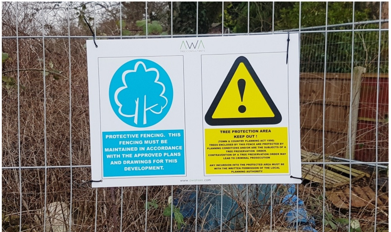
Figure 7: Example of A3 correx tree protection warning sign fixed to fencing panel
