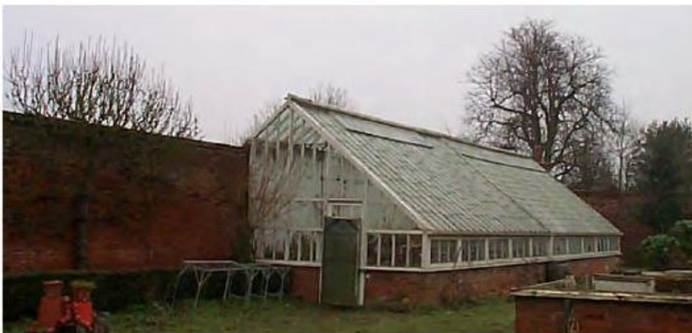
Figure 21a: Existing North wall building
