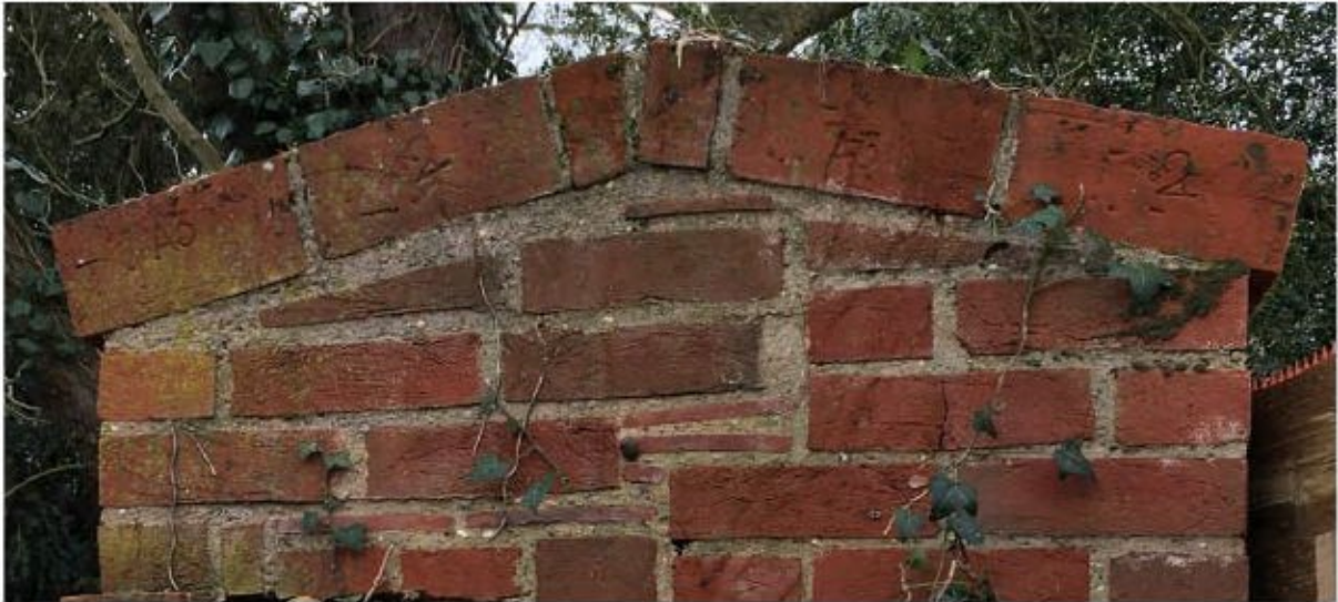
Figure 25: Capping to east end of South wall
