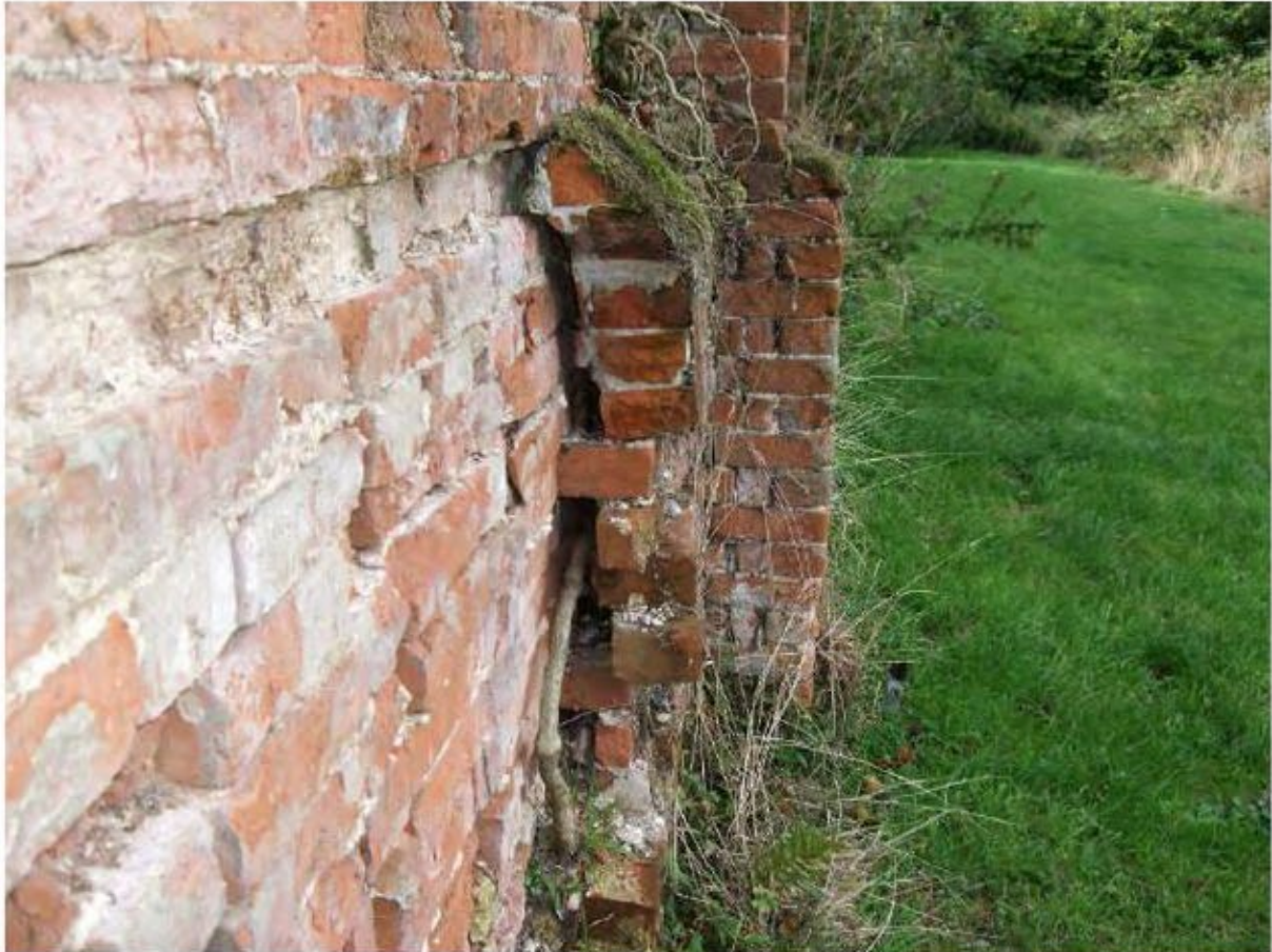
Figure 19: Delaminating plinth
