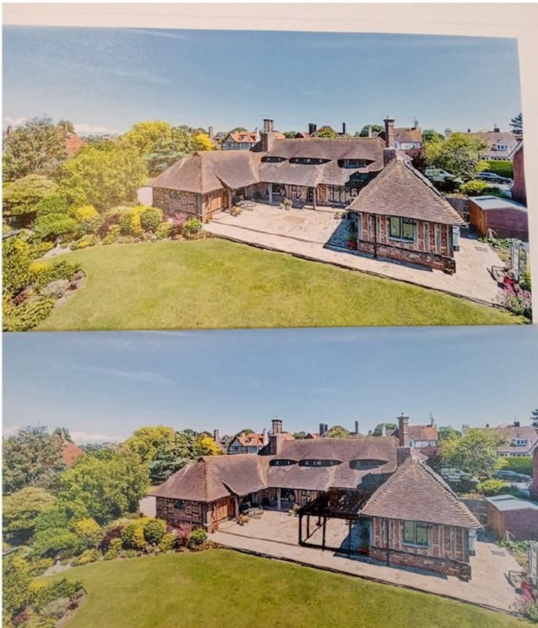
Aerial images showing the back of the house, and a black framed contemporary extension in the courtyard – discussed with Planning Officer.
