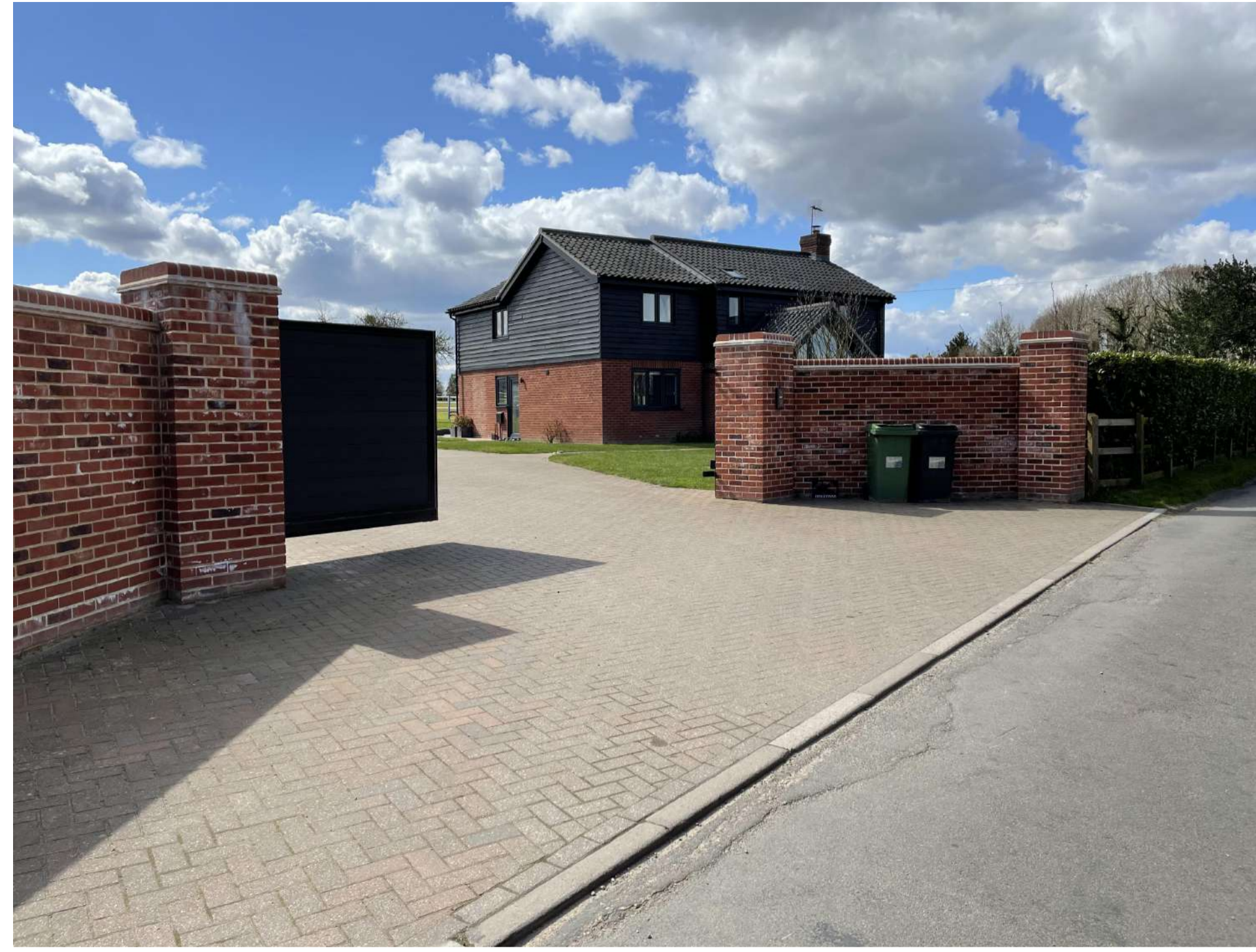
Image 02: Entrance viewed from East
