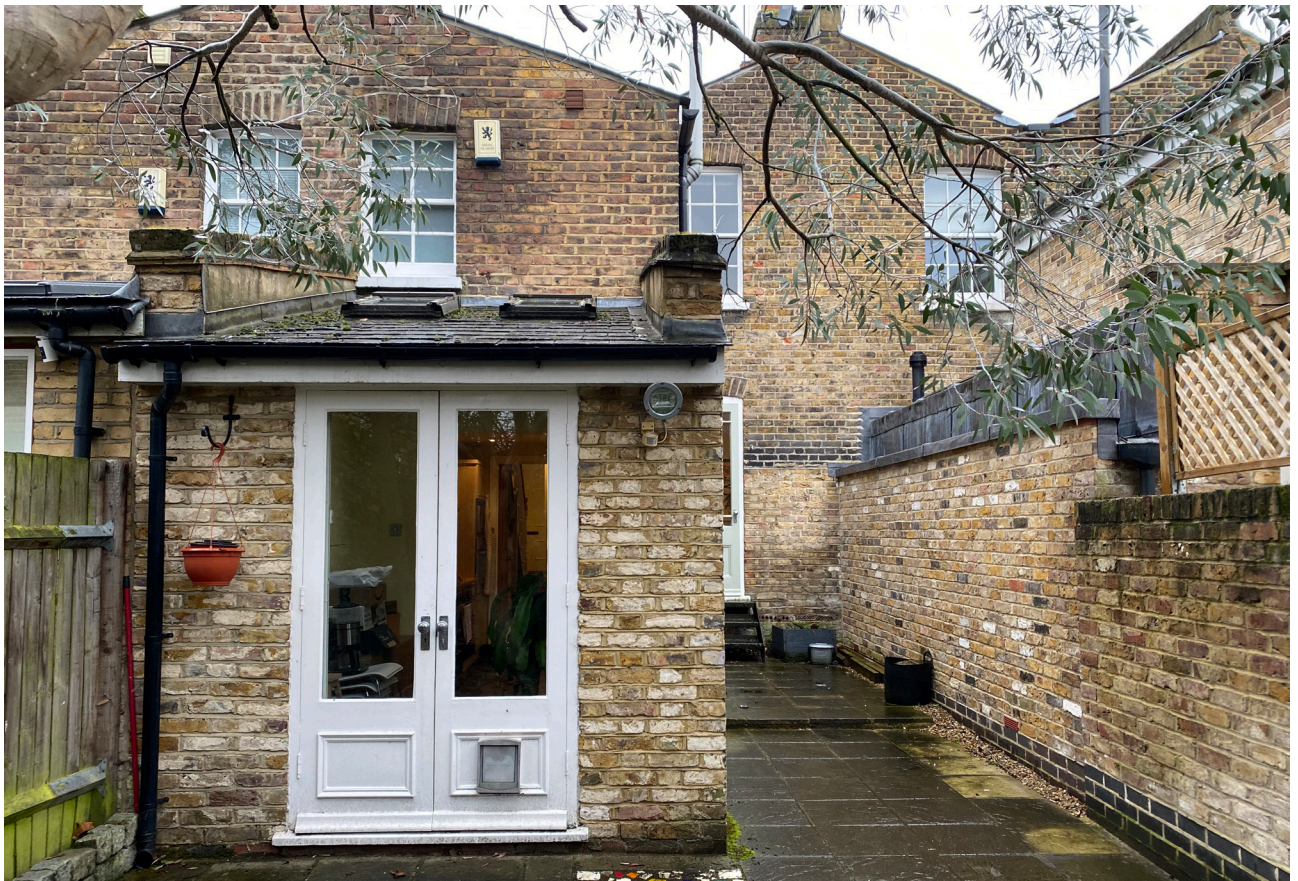
Existing rear elevation showing contemporary rear kitchen extension of 58, slightly higher rear extension of 59 (on left), and full-width, lead-clad side extension of 57 (on right).
