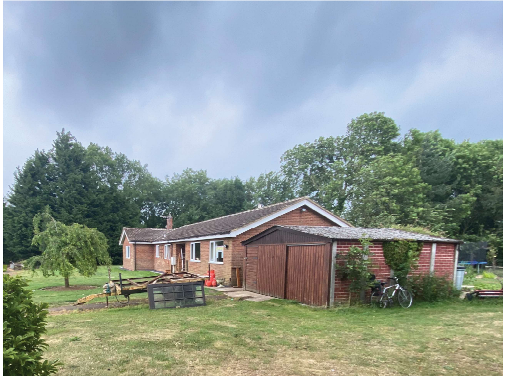
Right; Cedar farm, with garage to be demolished in foreground. New extension to be on this side of the existing building.
