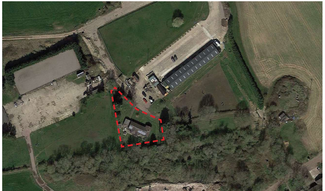
Right; aerial view of Cedar Farm, Cublington Road, Wing, Leighton Buzzard, LU7 0LB (site boundary highlighted in red dashed line)
