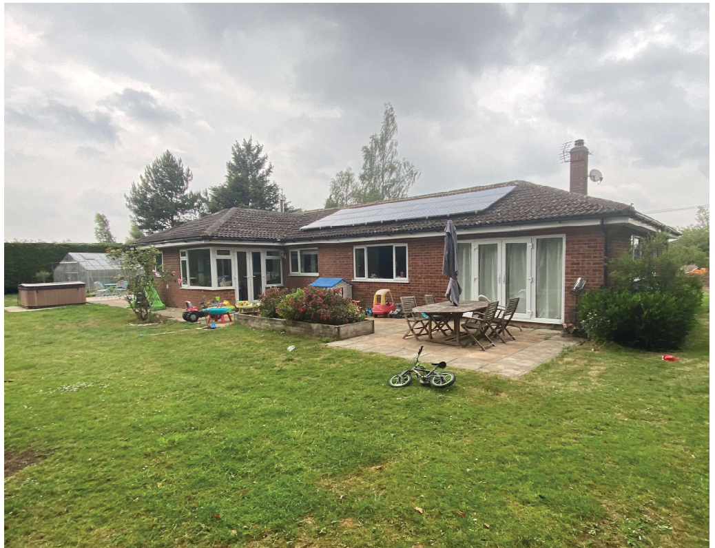
Right; Cedar farm from the rear of the bungalow.
