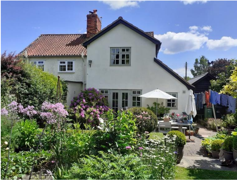
Fig. 3 - Rear elevation of the existing cottage
