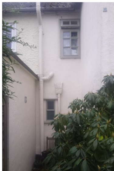
Fig. 4 - Existing ground floor window below bathroom currently blocked up
