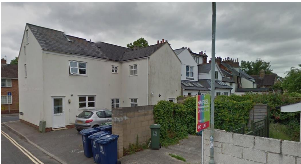
View towards 22 Vicarage Road – No.19 & 20's part single/part 2-storey extensions and no.20's loft dormer in the centre of the image.
