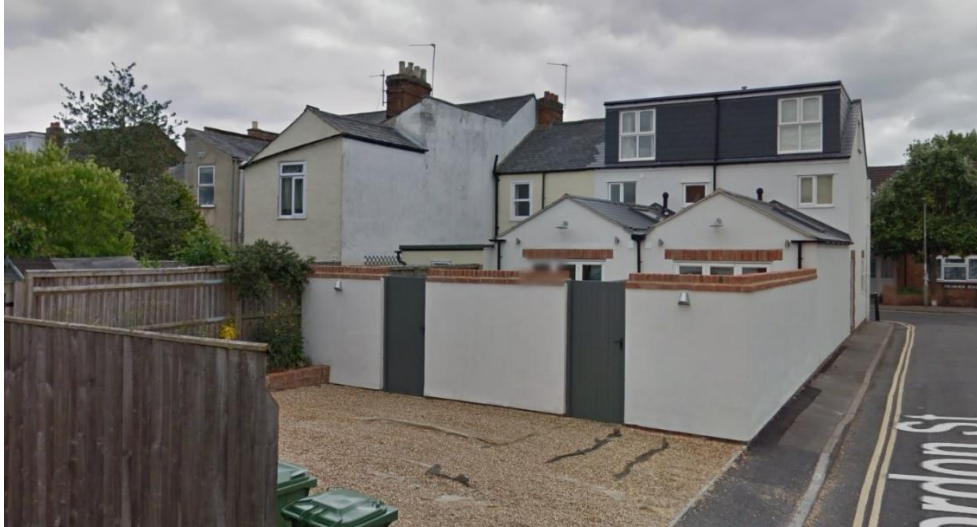
No.14 & 15's rear 2-storey extensions on the left of the photograph - No.16 & 17's part single/part 2-storey extensions and loft dormers on the right.
