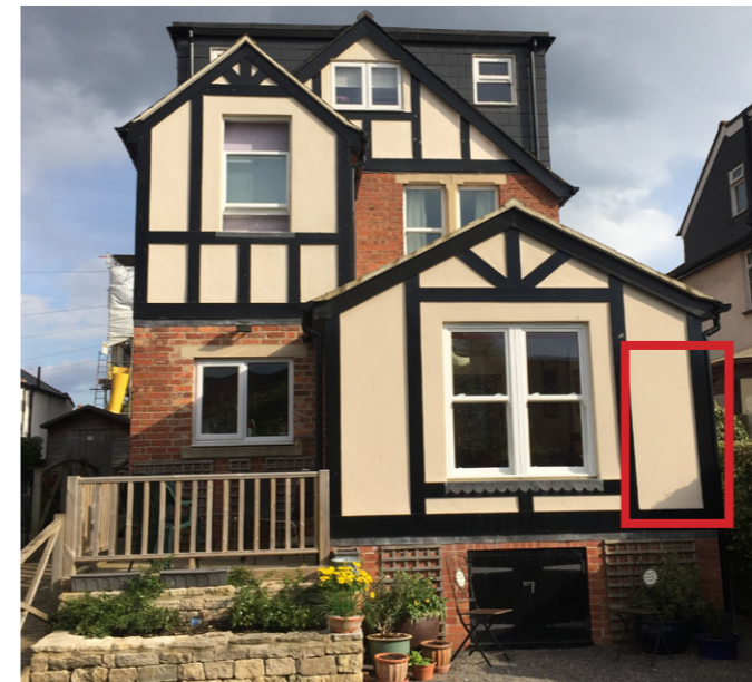
EXISTING REAR VIEW Showing proposed heat pump location
