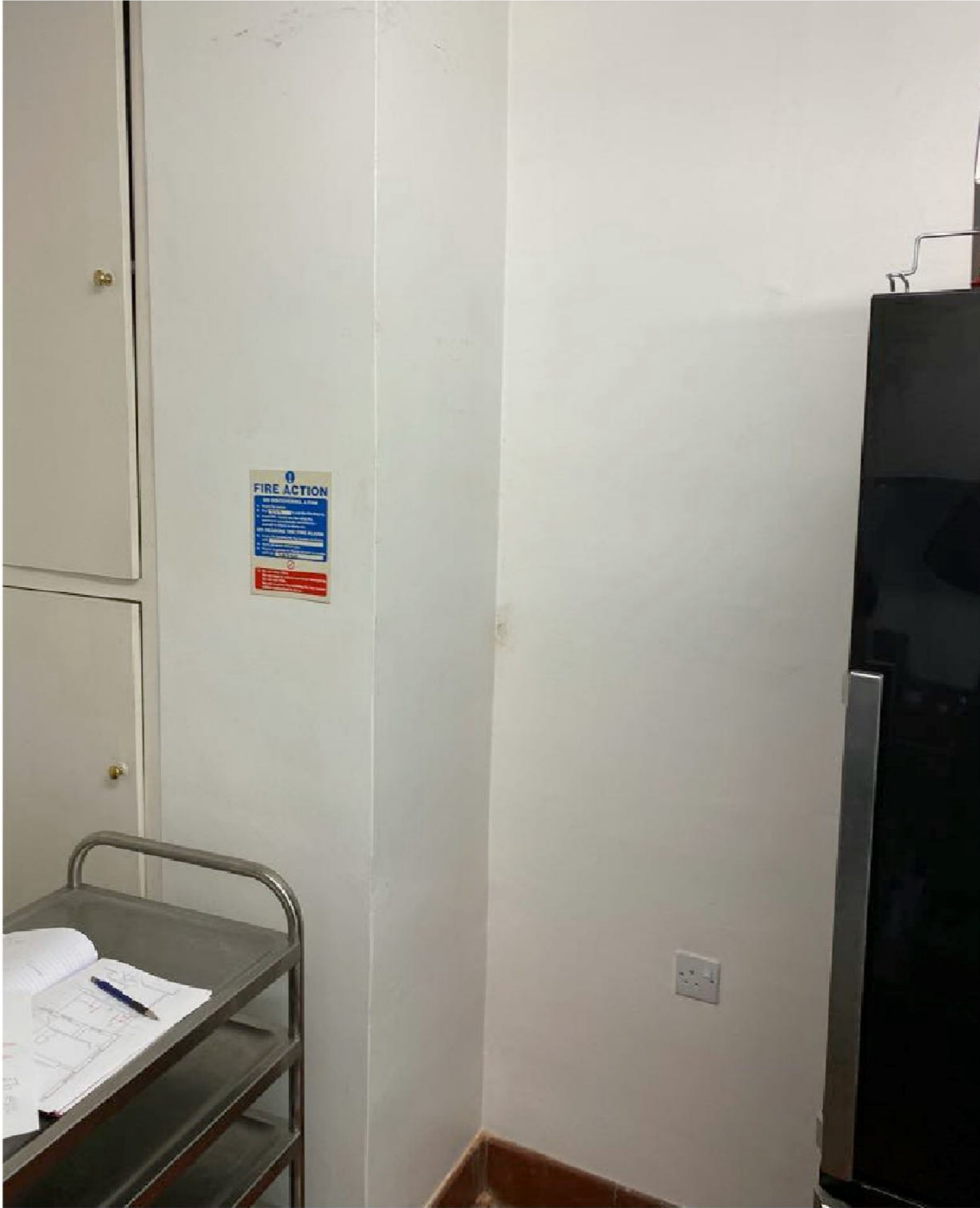
View within Canal House showing chimney breast which houses existing flue
