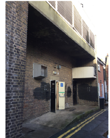
Figure 5 : View of the study site from High Street looking north.
