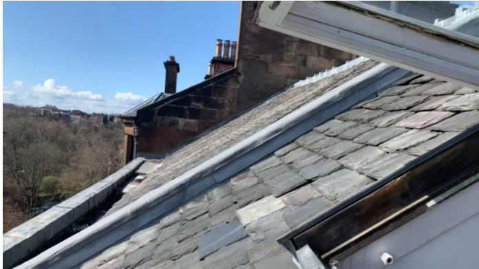
FIG. 2 VIEW FROM VELUX LOOKING NORTH WEST
