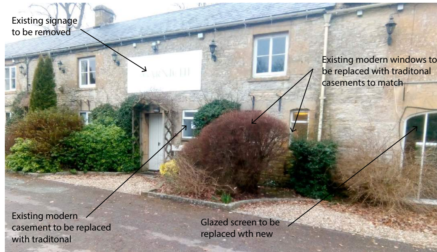
Photographs of modern signage and windows to be removed
