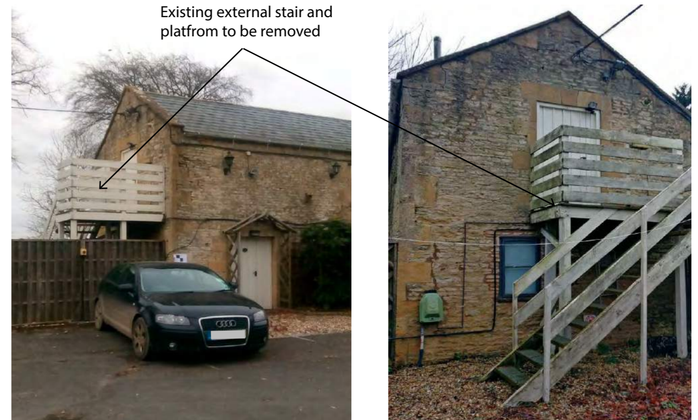
Photographs of existing external stair and platform to be removed
