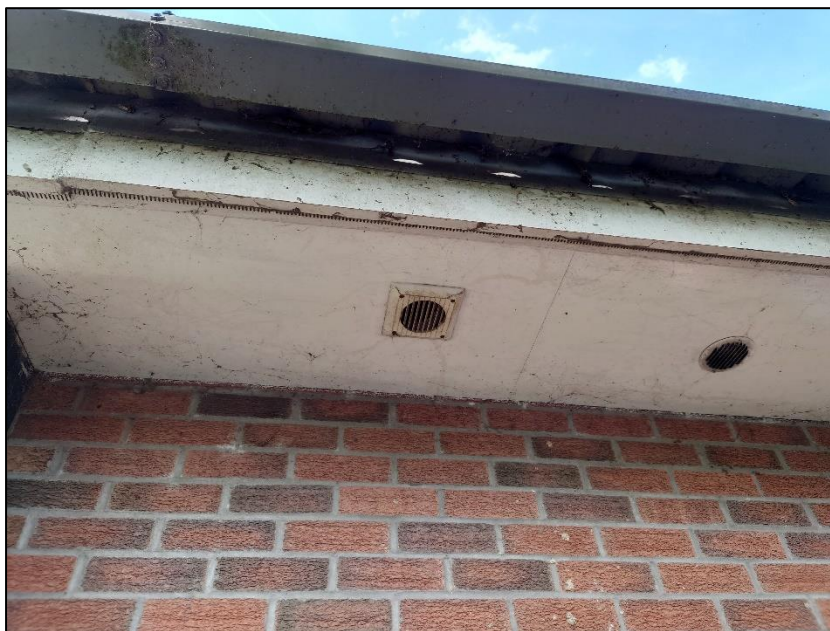
Photograph 3 showing peeling wood on the wooden soffit boards
