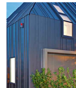
Metal faced vertical standing seam cladding Rheinzink - Private Residence
