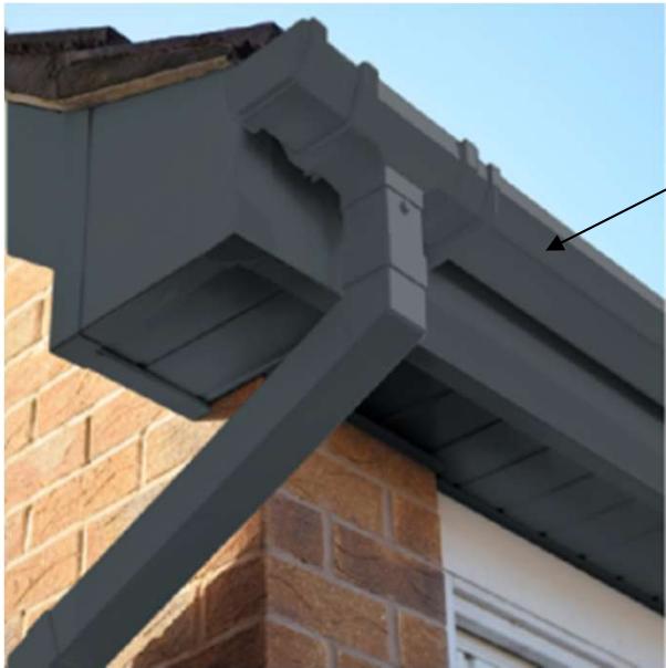
Gutters and downpipes
