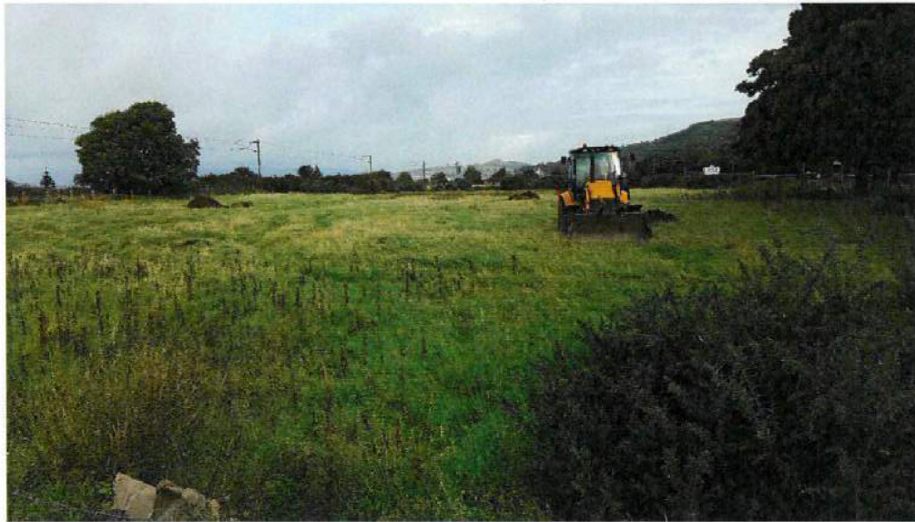
View North Across Site
