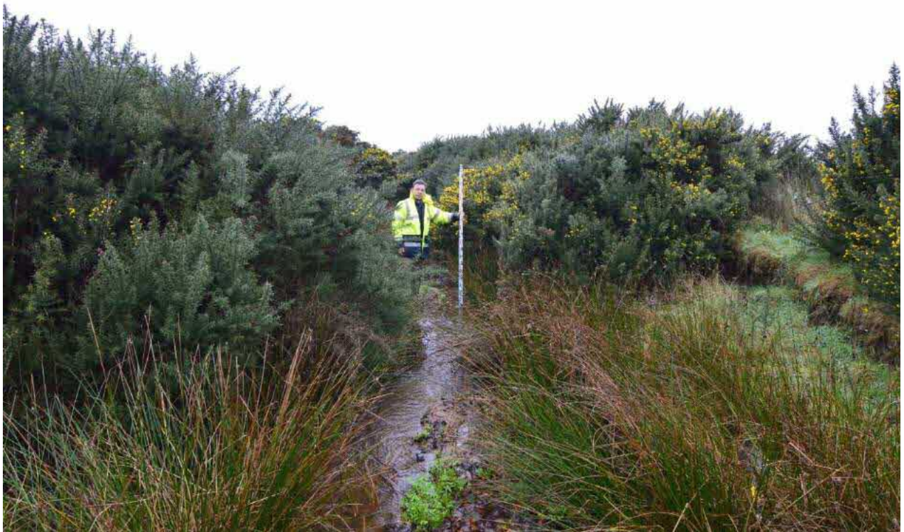
Plate 14: Channel of subject watercourse downstream of culvert outfall. Photograph taken from NS 21024 56293 looking downstream.
