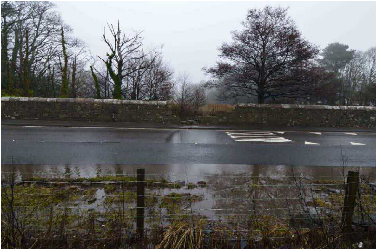
Plate 6: Looking east towards the source of the water pooling on the A78. The break in the wall was caused by a car crash. The field behind the wall is poorly drained and run-off flows onto the road. Photograph taken from NS 21039 56338.
