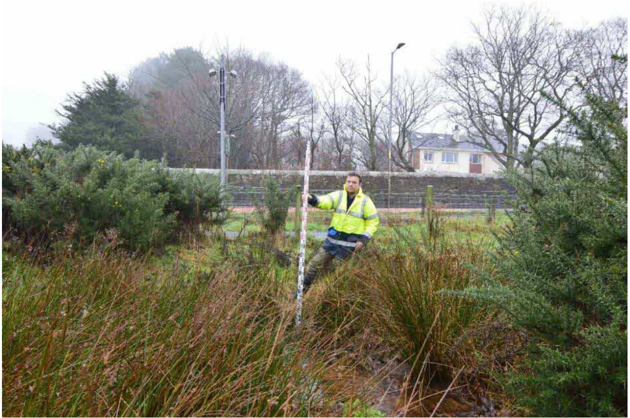
Plate 13: Channel of subject watercourse at culvert outfall. Photograph taken from NS 21018 56294 looking upstream.
