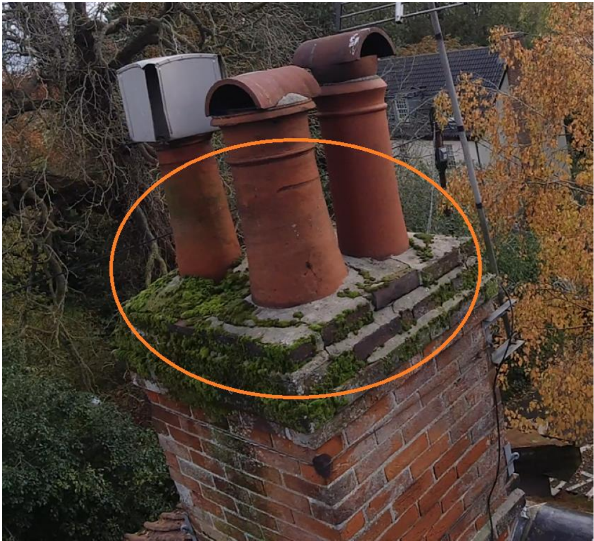
The concrete cap to the top of the main chimney stack.
