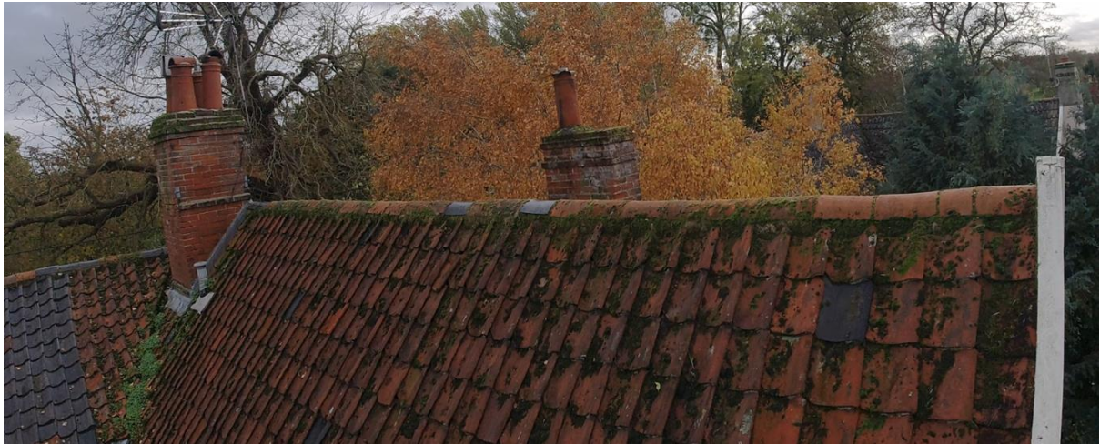
A view of the rear roof.
