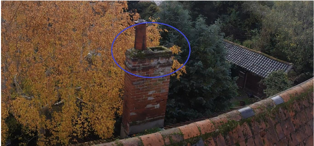
The rear chimney stack, with an open flue.
