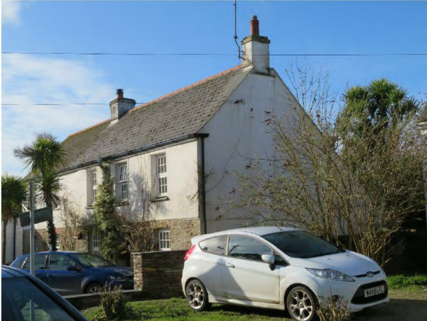
Photo 1 Existing north gable wall
