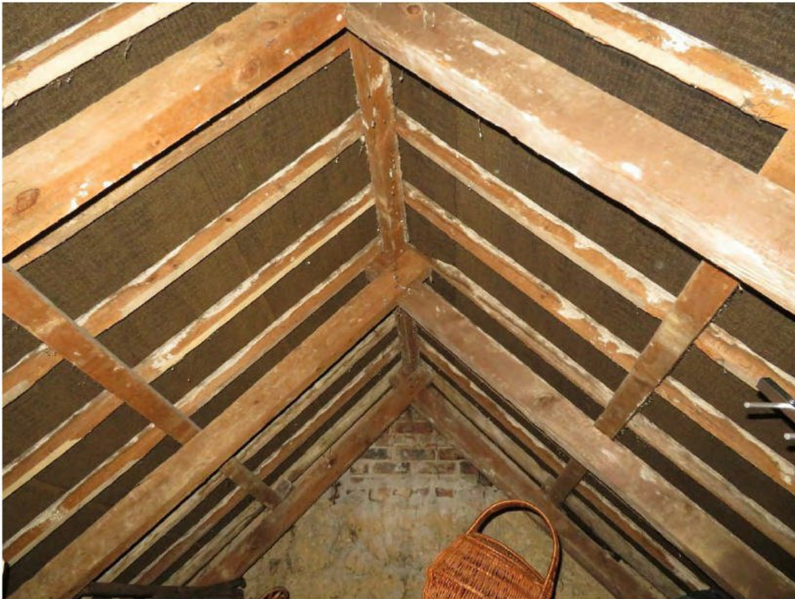
Photo 5 Internal view of north gable wall and roof structure
