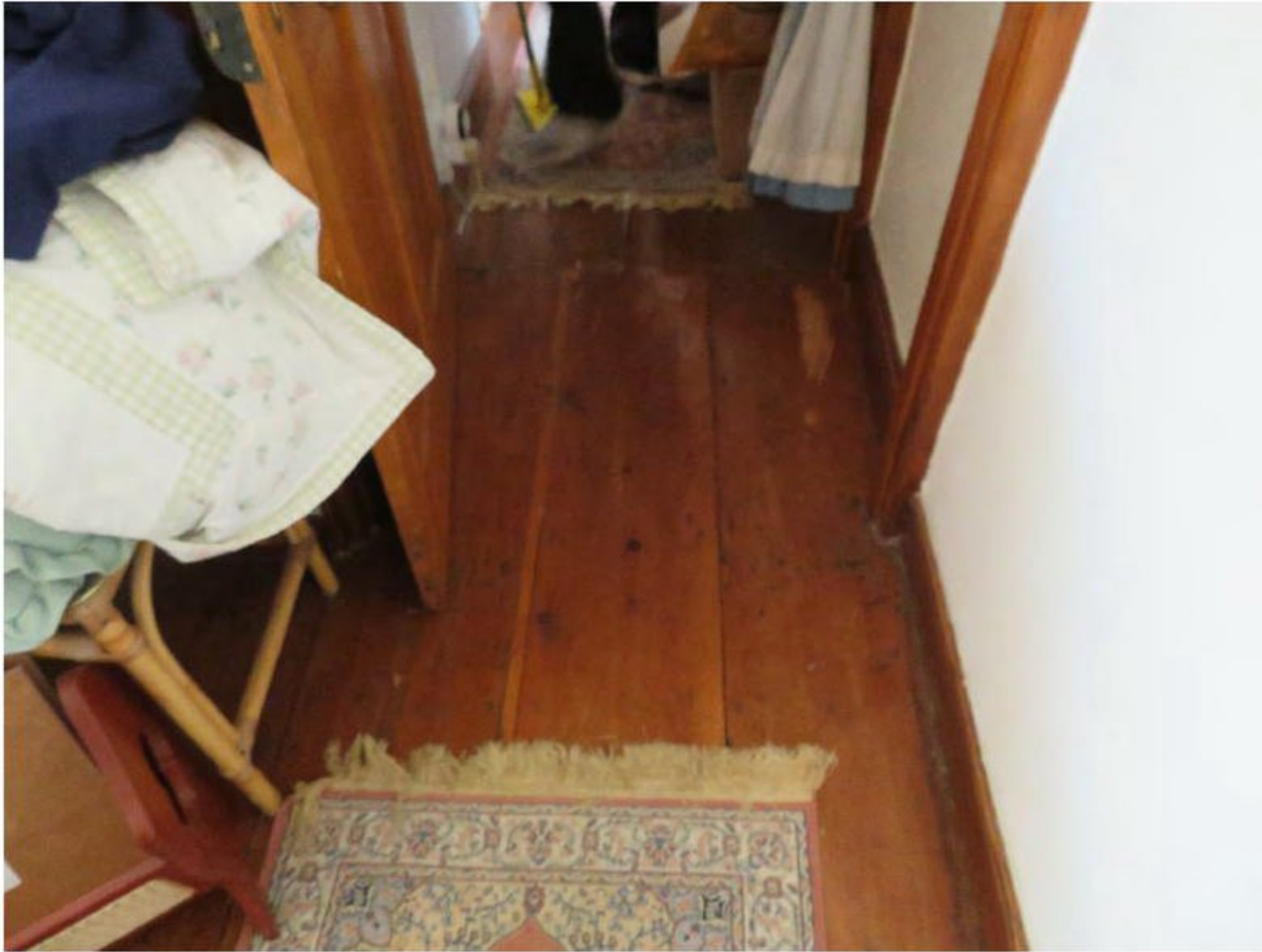
Photo 7 Existing floorboards at northern bed room parallel to length walls
