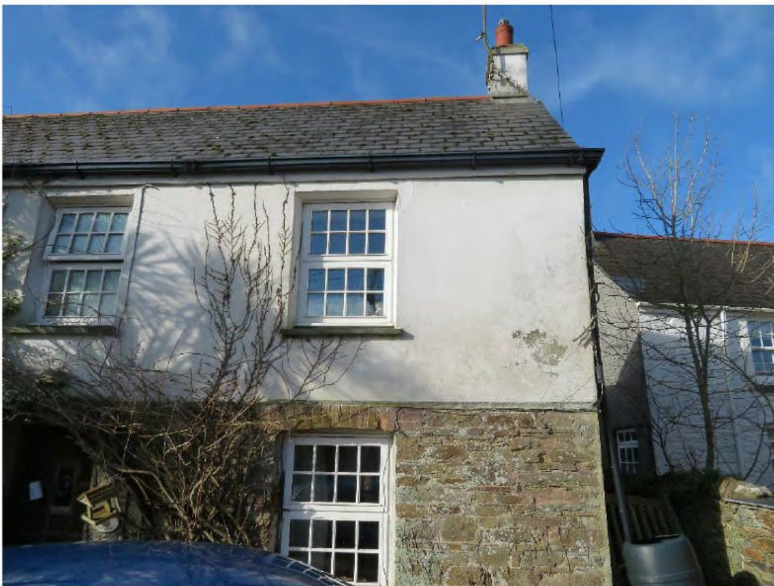
Photo 2 Northern section of east (front) elevation
