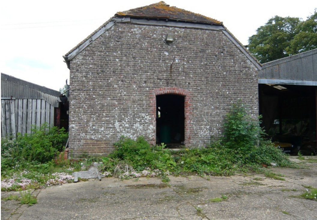
Photo 2 Barn/granary east elevation with bricked up cart entrance to Bay 3
