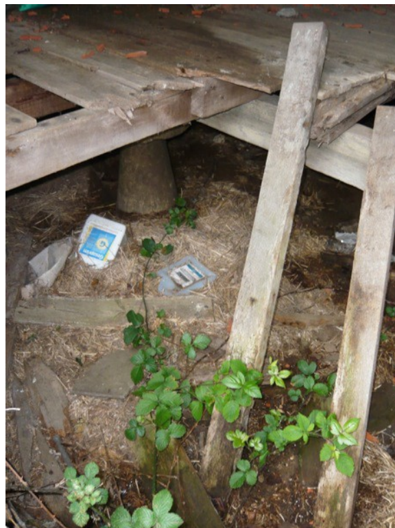
Photo 4 Machine sawn timber floor construction
