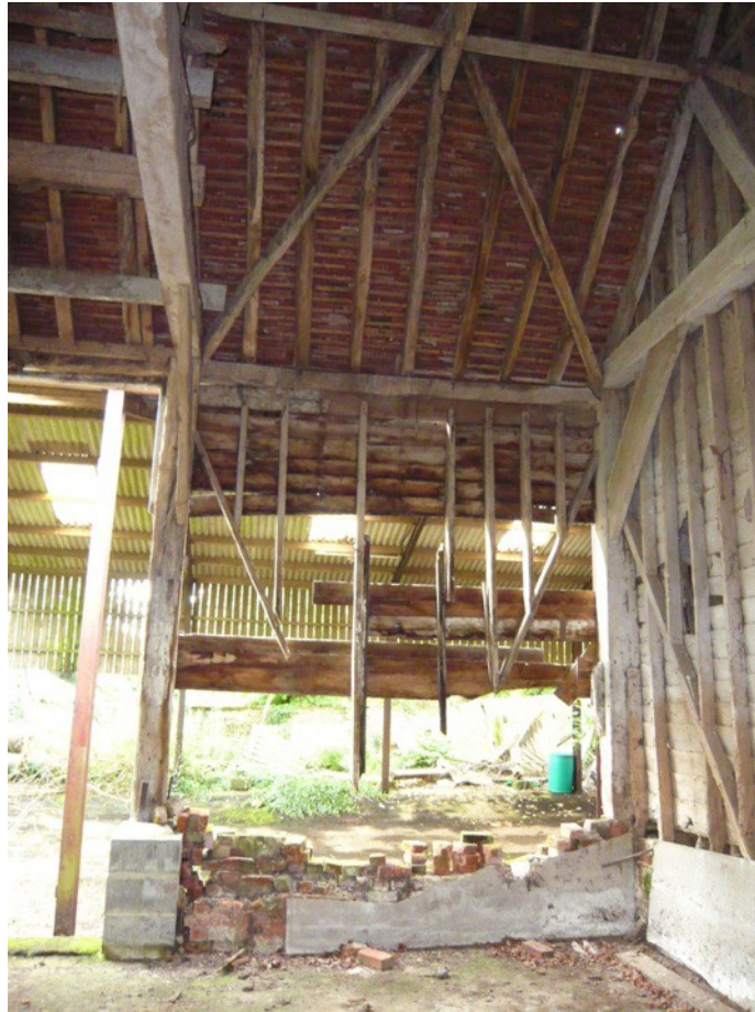
Photo 8 Dairy building King post roof trusses
