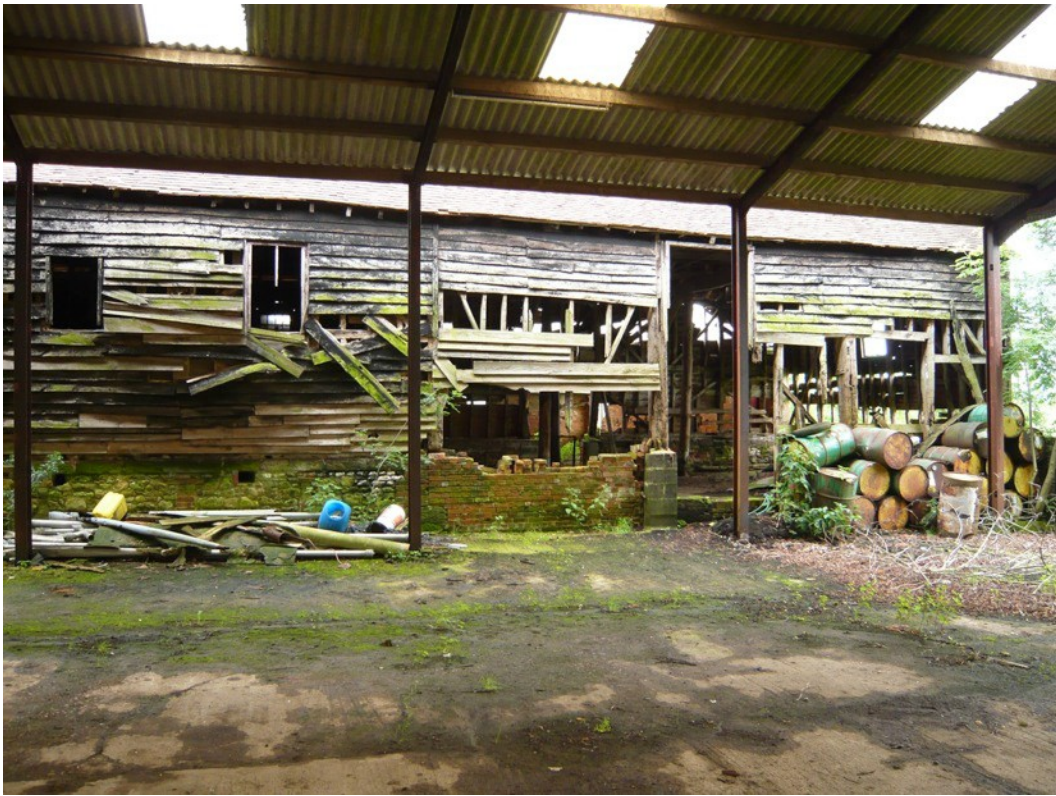
Photo 4 Barn/granary west elevation with bricked up cart entrance to Bay 3
