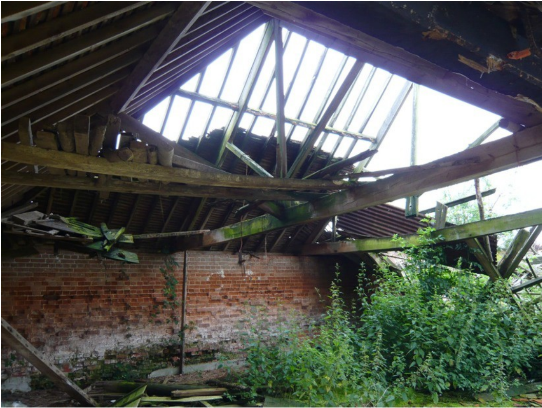
Photo 10 Southeast cartshed wide span King post roof truss
