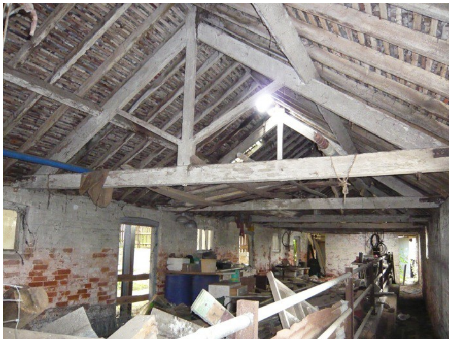
Photo 8 Dairy building King post roof trusses
