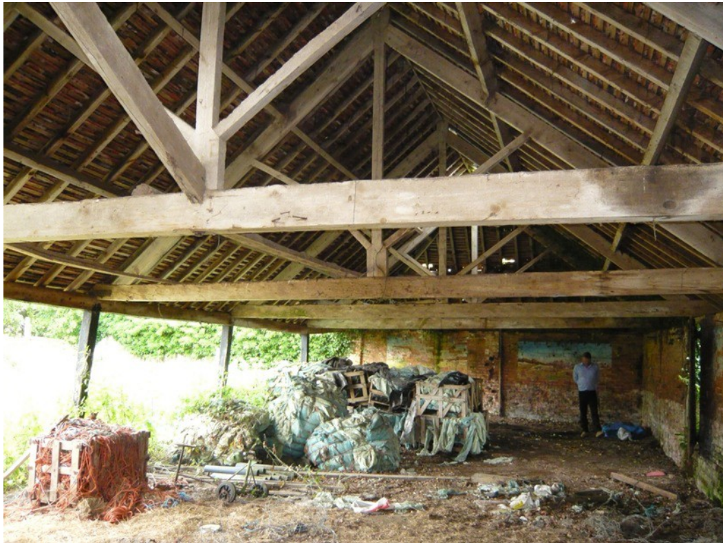
Photo 10 Southeast cartshed wide span King post roof truss
