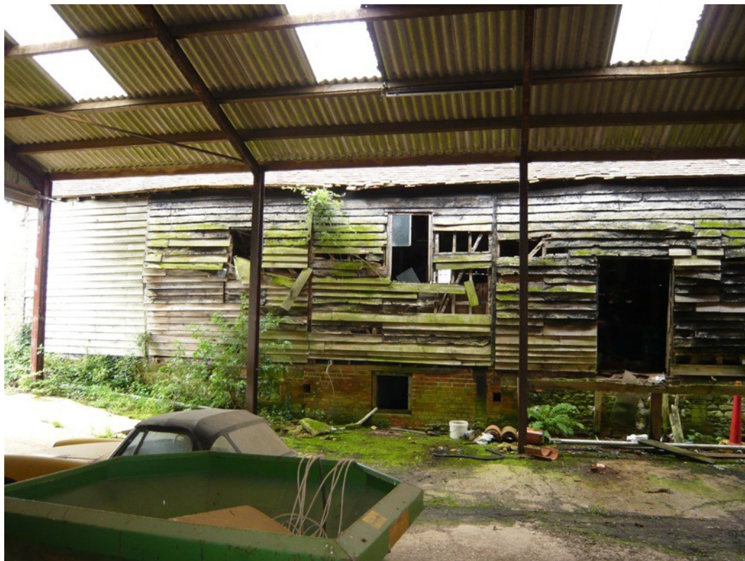
Photo 2 Barn/granary east elevation with bricked up cart entrance to Bay 3
