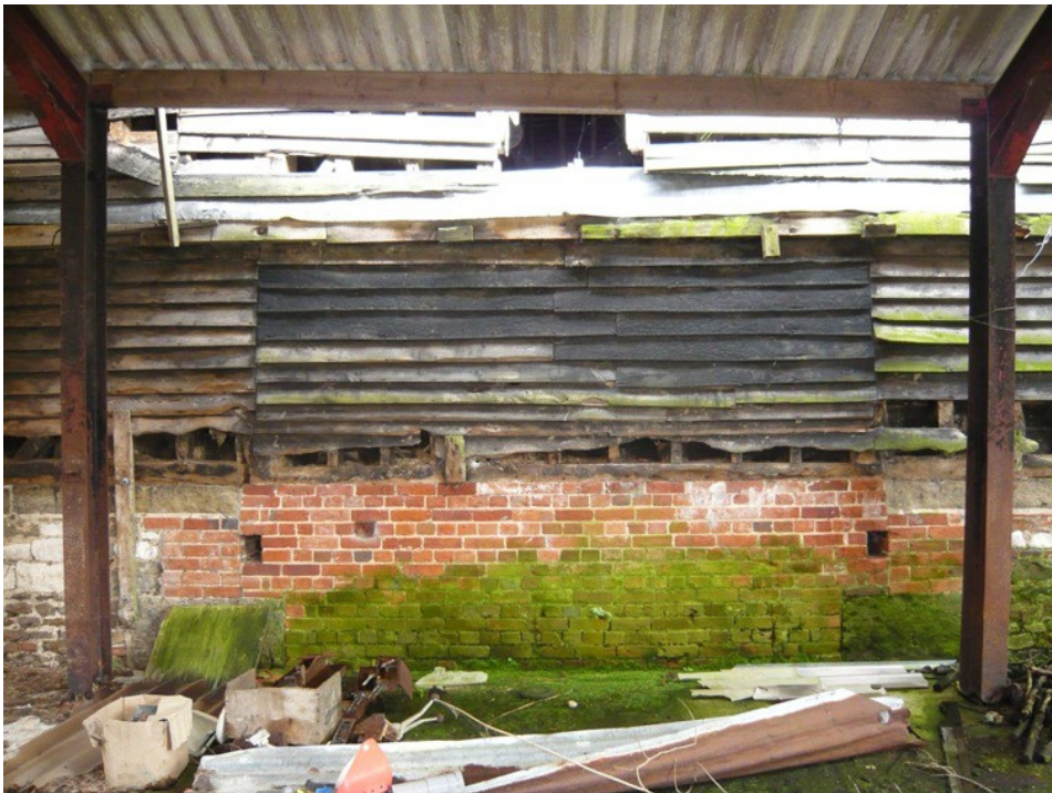
Photo 4 Barn/granary west elevation with bricked up cart entrance to Bay 3
