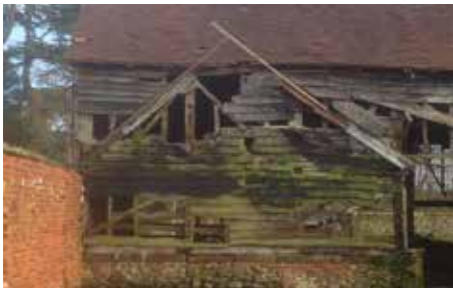
Photograph showing the original link building zinc flashing
