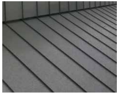
Pre-patinated standing seam zinc roof
