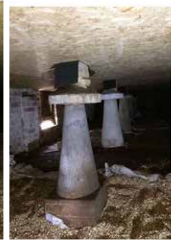
Original saddle stones present in bays 1 - 3
