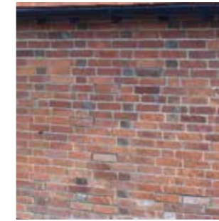
Existing brick wall
