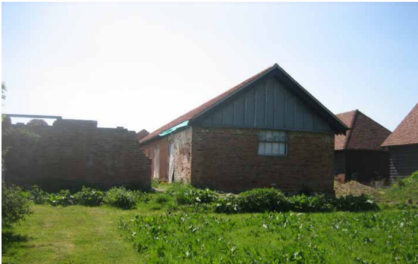
Photo taken by the Client looking South towards the Dairy Shed.
