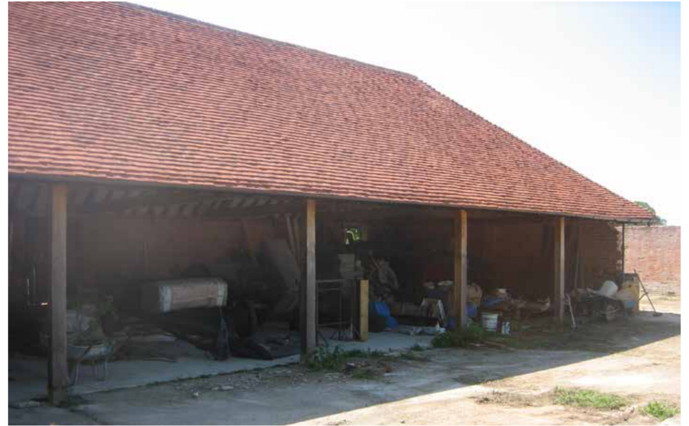
Photo taken May 2020 of the repaired Machine Shed
