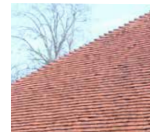
Existing roof tiles
