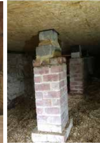
Brick Piers more recently added
