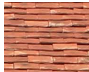
Recycled tiles from site
