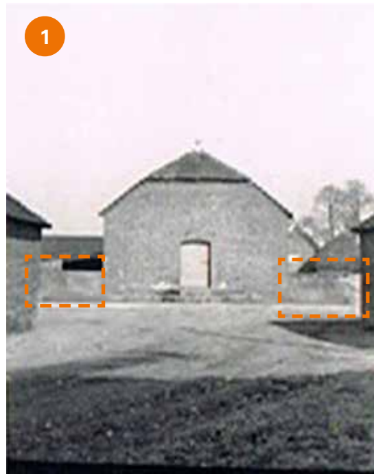
Historic photograph of the Granary gable wall showing the extent of the adjoining brick and stone wall
