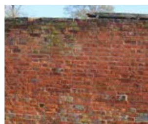
Brick wall from recycled bricks from site
