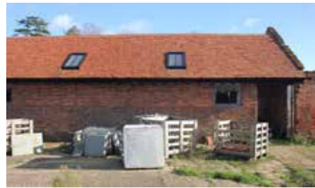
Photograph showing the current status of the Dairy roof
