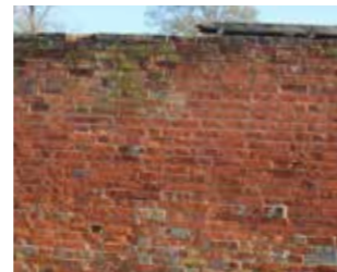
Brick wall from recycled bricks from site
