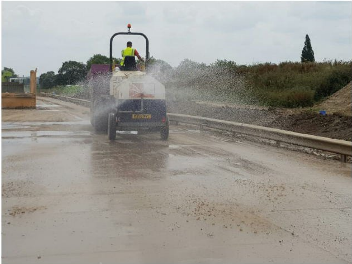
Use of water bowser for dust suppression on site roadways
