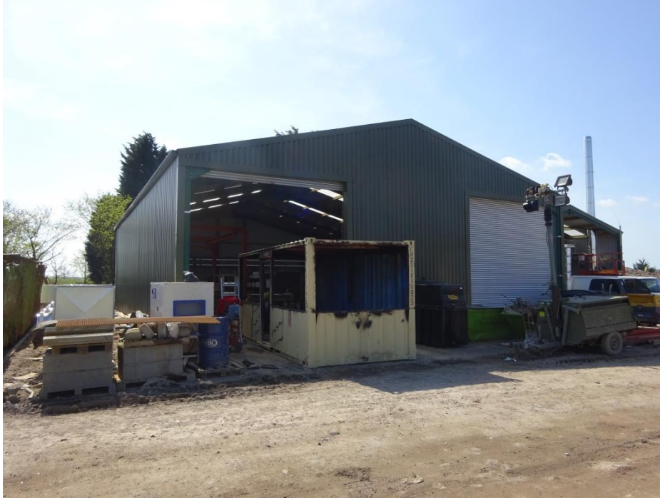
Fully enclosed workshop (Door open as staff working on large machinery)
