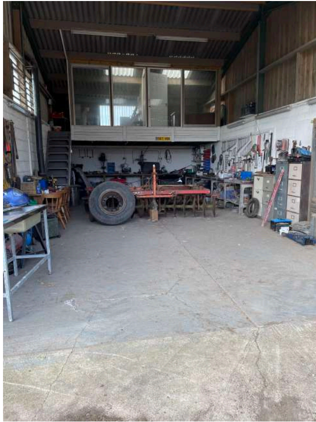
Photograph 11 (Farm Machinery Maintenance Workshop)
