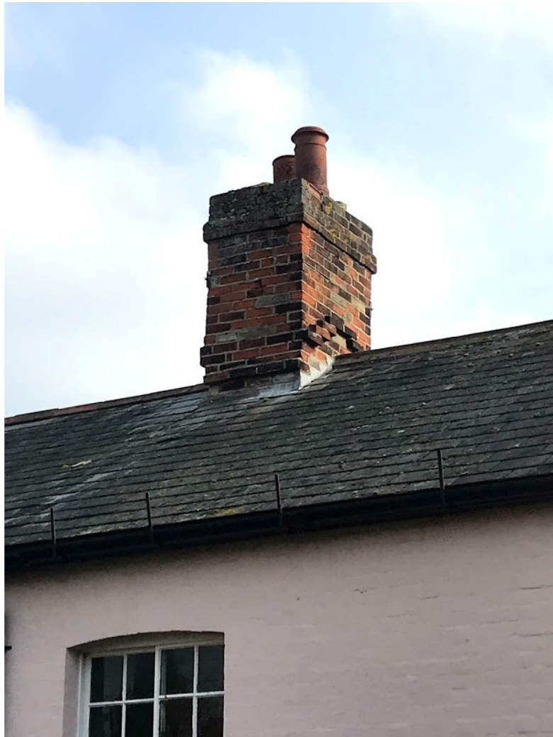
View of chimney from West
