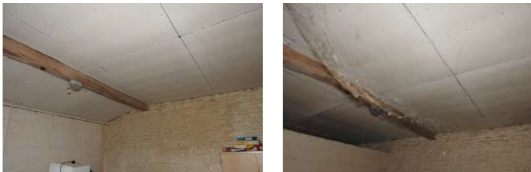
Figs. 9 & 10 Hardboard lined ceiling of the stables
