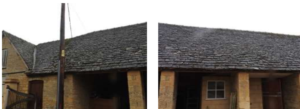
Figs. 5 & 6 Ridges and roof tiles to the front
