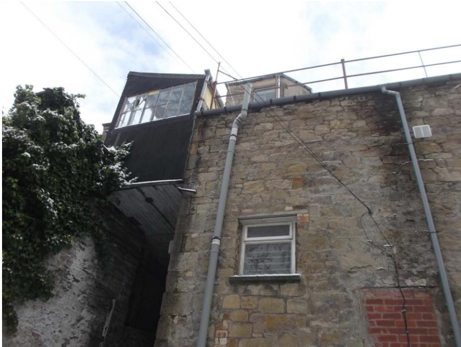
Photograph 1 – View of northeast elevation
