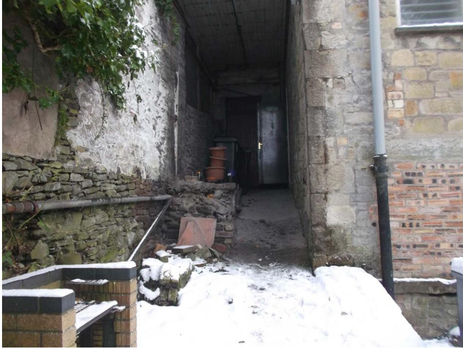
Photograph 6 – existing ramp & fire escape
