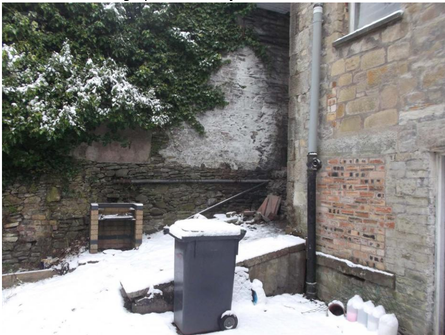
Photograph 2 – View of northeast elevation and existing ramp
