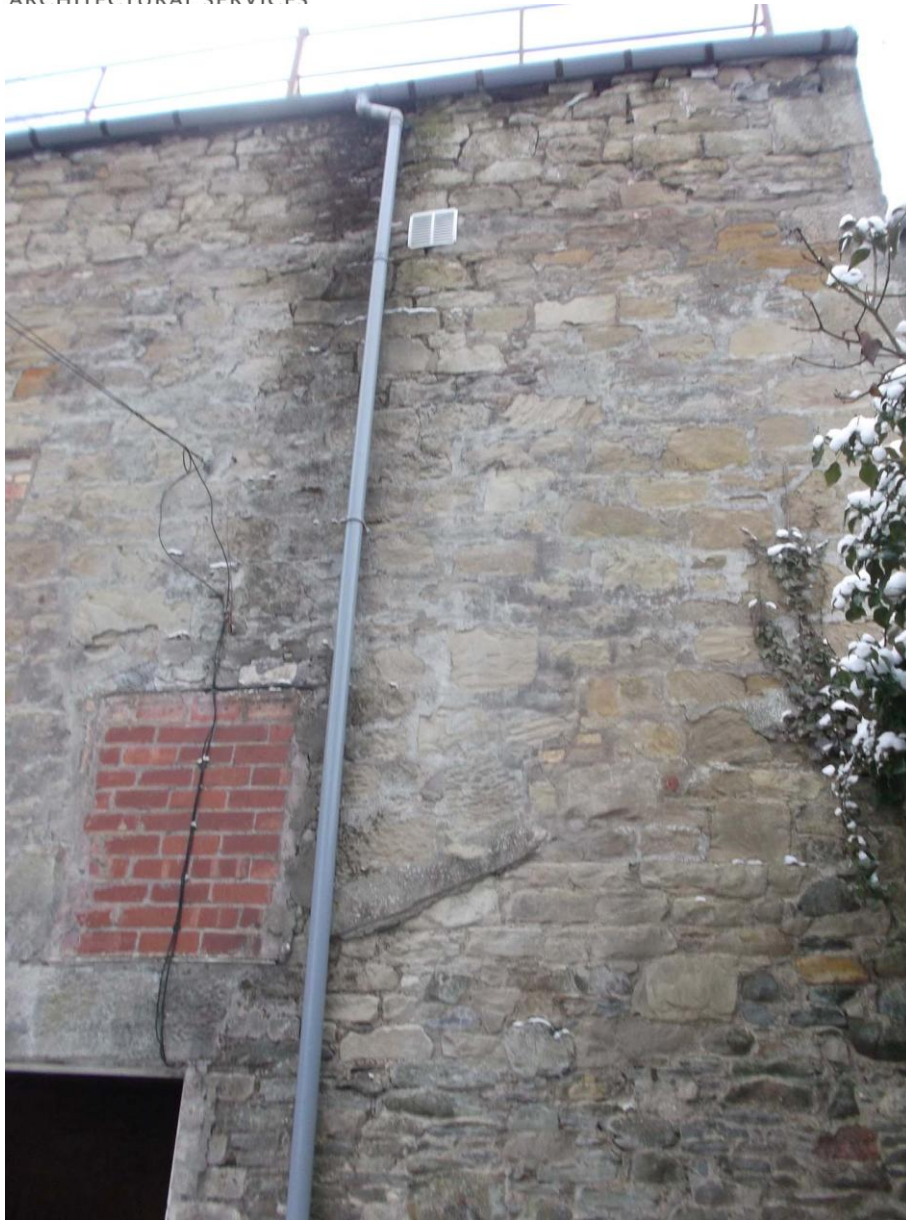
Photograph 5 – view of northeast elevation (blocked opening visible)
