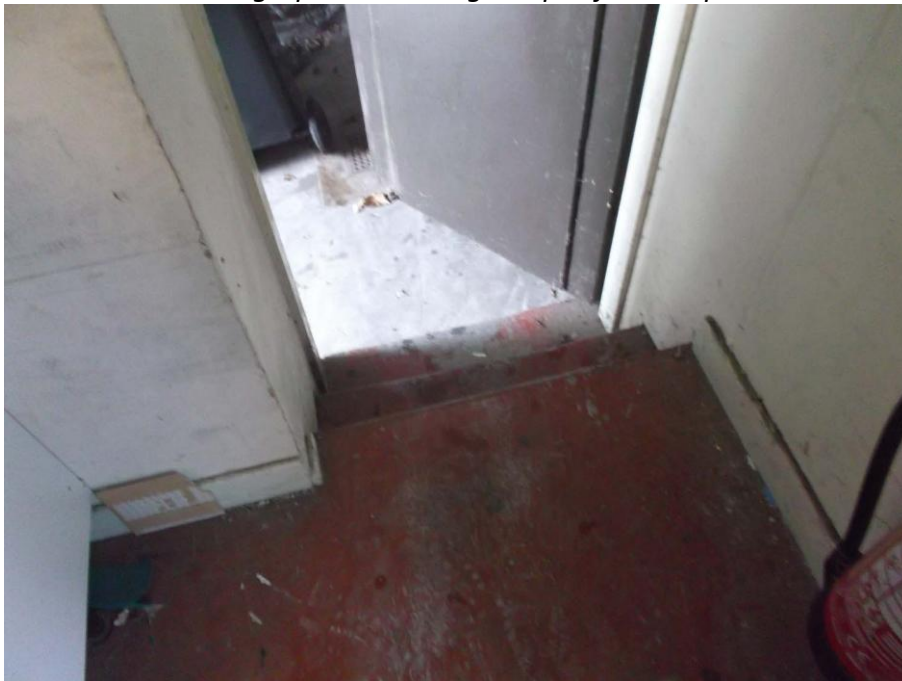
Photograph 7 – existing fire escape steps to be altered.
