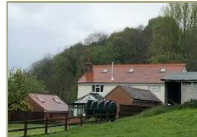
Image 4: South west elevation of Sunnybank Cottage
