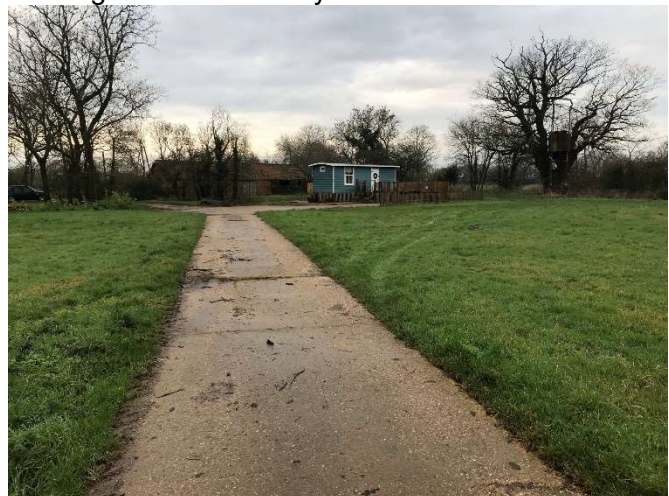
Existing Access Driveway from Unit 6 to Unit 8
