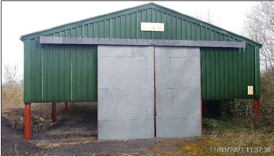
Figure 1a: South western elevation of B1.
