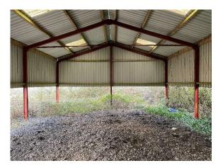
Generally it is in good condition apart from some minor corrosion to the steel columns but this is considered to be surface only with negligible loss of cross-section that would affect structural integrity.
