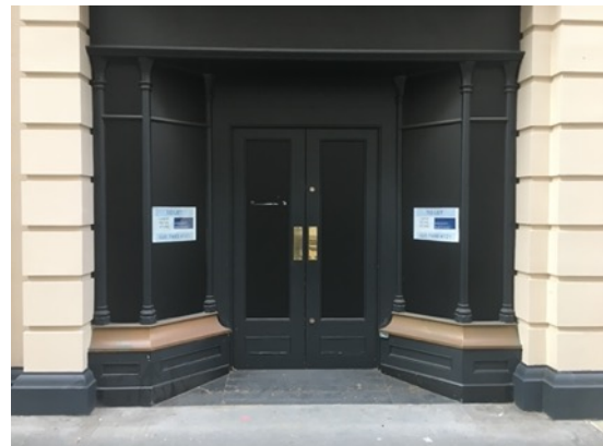
Existing Unit 3 entrance, which will remain unchanged
