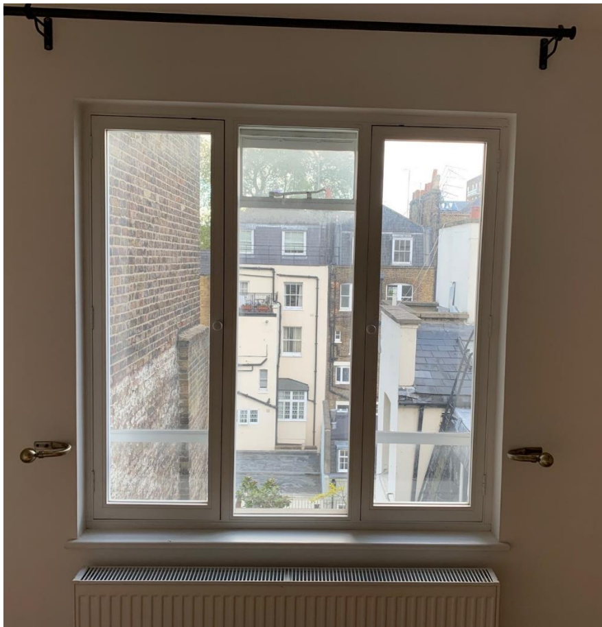
Photo sheet no.3 – New secondary glazing detail to Bedroom 2 W.06
