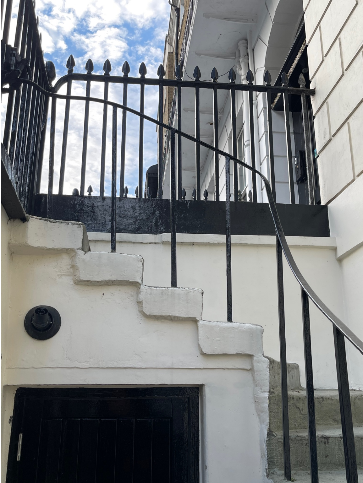
View of steps and handrail
