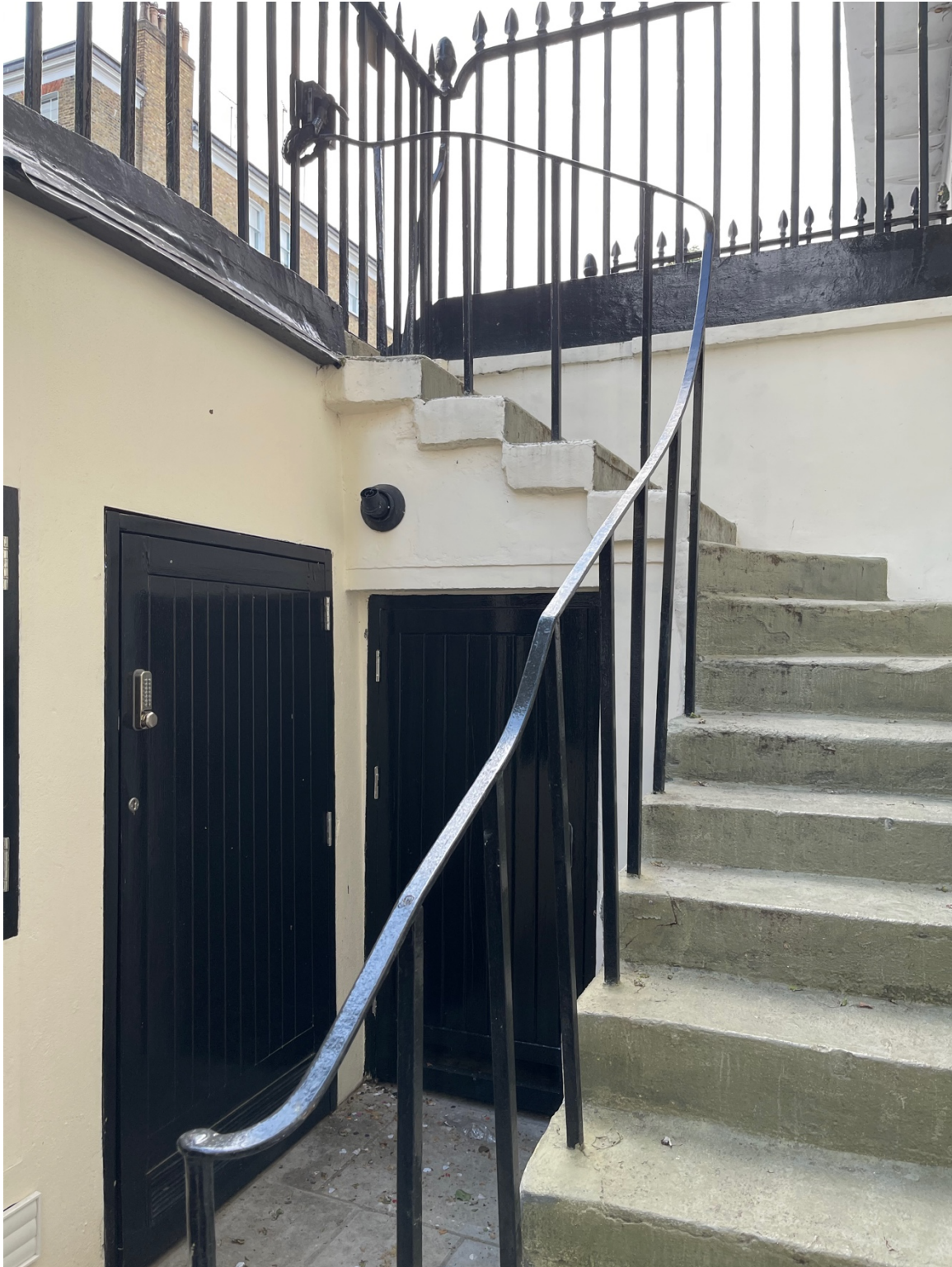
Another view of the steps and handrail
