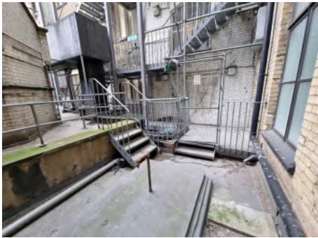
EXISTING PHOTOGRAPHS OF PLANT AREA
