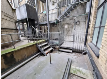
EXISTING PHOTOGRAPHS OF PLANT AREA
