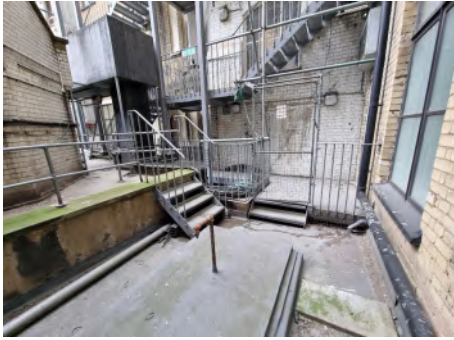
EXISTING PHOTOGRAPHS OF PLANT AREA
