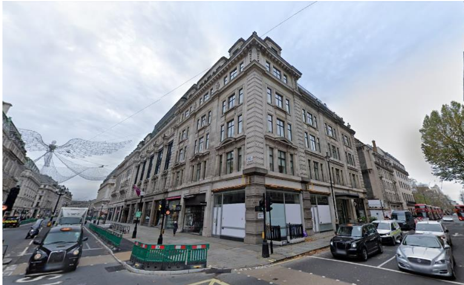
Figure 1: Image of the front elevations of the Site
