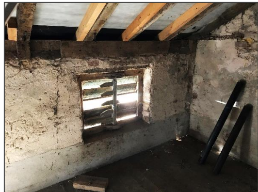
Photo 8: Open vent on upper floor.
