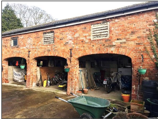
Photo 1: West aspect, open archways.
