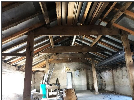
Photo 7: Upper floor internal construction.
