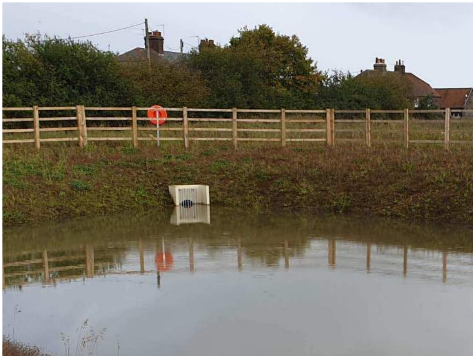
Plate 8: Slight drop in water observed 6 hours after Plate 7 was taken. There was no rain in these 6 hours.
