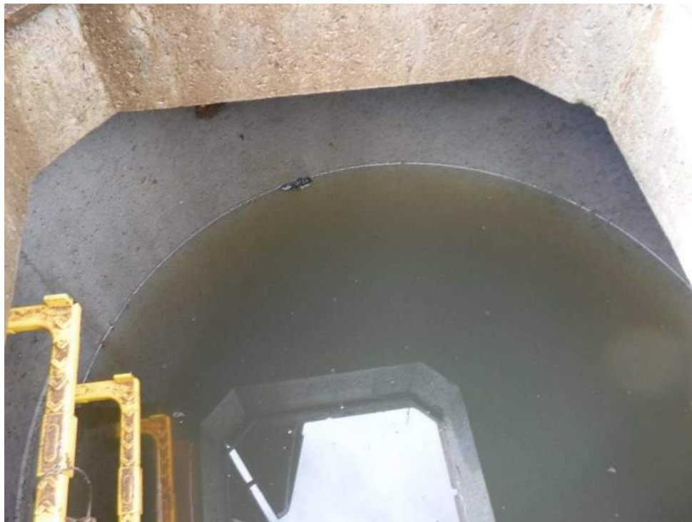
Plate 4: Hydrobrake chamber on 8 th October 2020.
