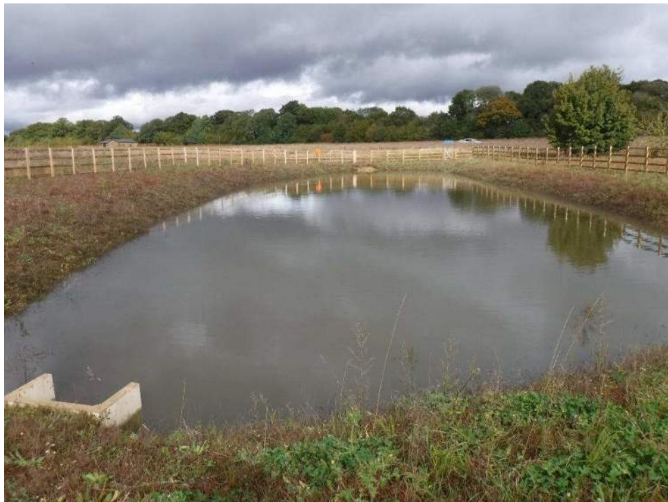
Plate 6: Attenuation pond on 8 th October 2020.
