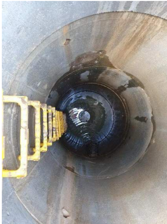
Plate 1: Borehole soakaway on 29 th September 2020.
