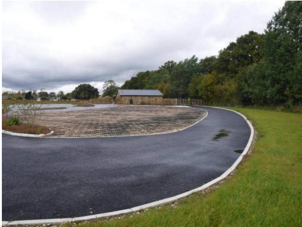
Plate 5: Existing area of permeable car parking.
