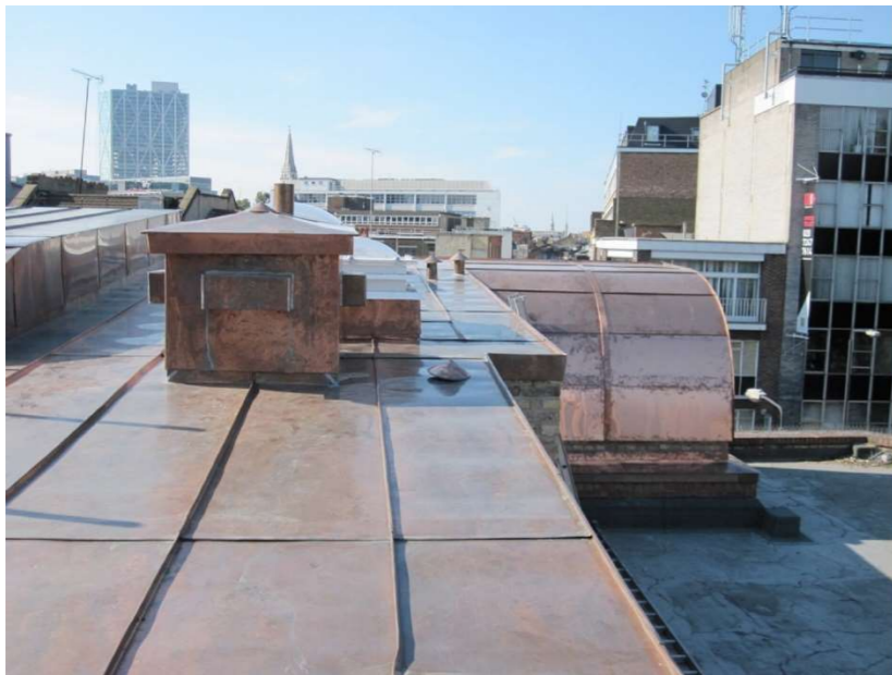
2010: Part of the new copper roof.
