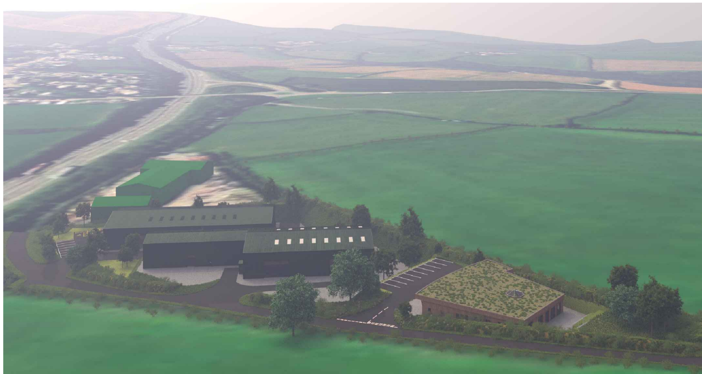
SITE VIEW LOOKING TOWARDS THE SOUTH WEST
