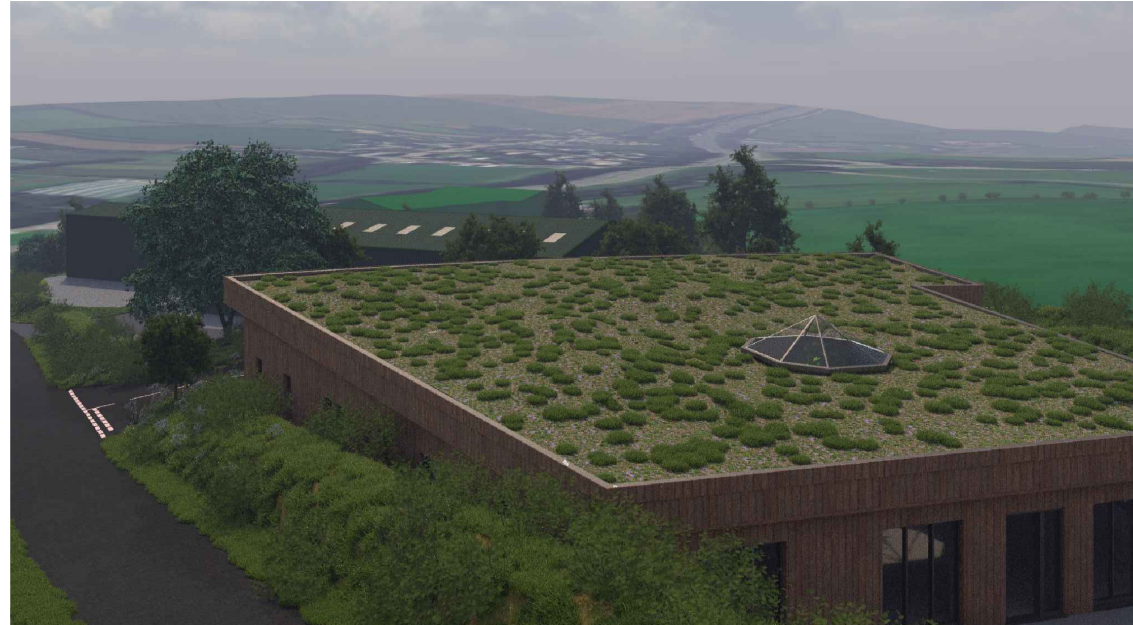
SITE VIEW LOOKING TOWARDS THE SOUTH WEST
